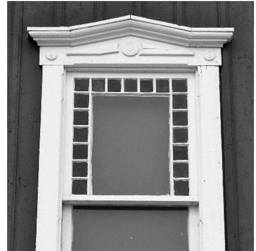
FIGURE 3. The depot’s colored glass window. Square panes of colored glass border the upper frame of a second story window where the stationmaster lived. Photo by J. Carl, June 2009.
