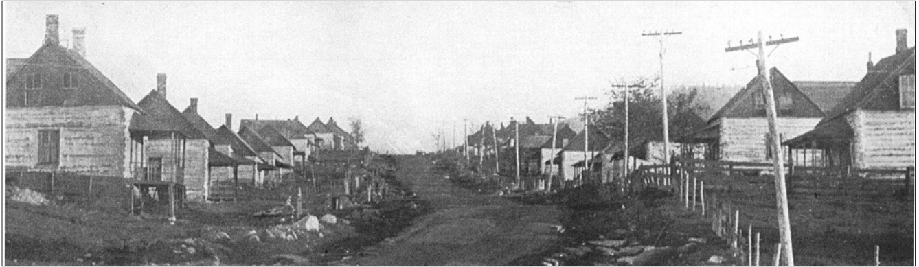
FIGURE 5. “Log cabins” in a mining camp that was not Jayville. The houses were built for employees of the Chateaugay Ore and Iron Company along a dirt road at Lyon Mountain in Clinton County. Only the walls were made of logs, whereas boards were used in the upper story and front porch. Reproduced from an 1885 photograph in J. R. Linney, 1934, p. 47.
