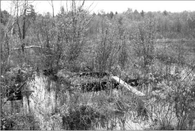
FIGURE 14. Concrete pilings and the square foundation of a railroad water tower. The circular interior is reached by a board. See sketch map of the railroad yard for location (Fig. 11). The water tower was removed after 1920. 25 Photographer James Carl stood on the tracks.
