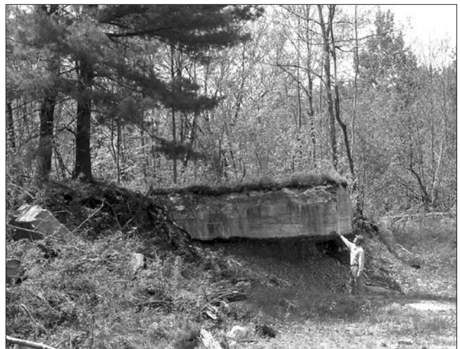
FIGURE 19. A thick slab of concrete protrudes from the edge of a recent gravel pit. Underlain by sand and boulders, the slab once was level with the surface. Concrete pilings on top suggest that it may have supported a mine building, an ore crusher or a loading platform for railroad cars parked on a spur. Photo by J. Carl, May 20, 2009. Bill Mueller poses for scale.
