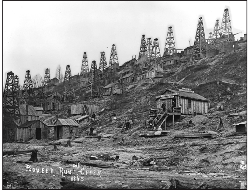
FIGURE 12. High density oil well drilling. A hillside at Pioneer Run near Oil Creek, northwest Pennsylvania, in 1865. The shack (right center) has signs reading "Shoe & Leather Petroleum Co, David Harris, Supt.," and "E. C. Bishop, Act., Foster Farm Oil Co." Ten men and two seated, well-dressed ladies posed for the photographer. Note the tree stumps in the lower left. Imagine the muddy quagmire created here during a heavy rainstorm. The photo, reproduced from the collection of the Drake Well Museum, was purchased by James Carl in 1993.
