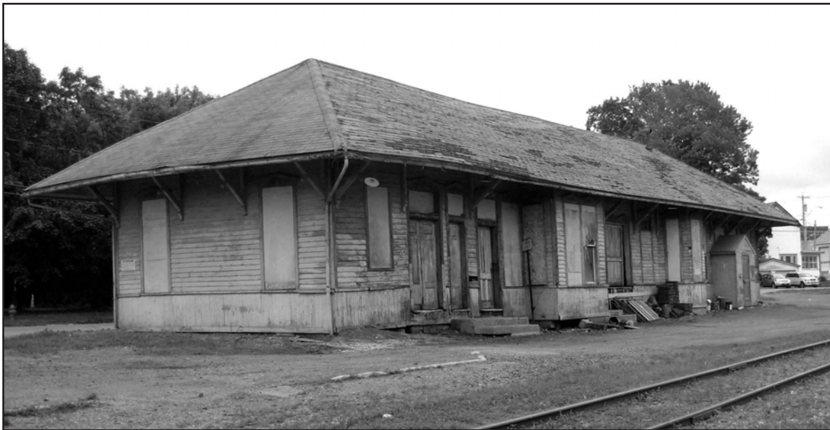
FIGURE 17. Still standing in downtown Carthage is the 1884-1885 New York Central passenger depot on North Mechanic Street, erected after the city fire of 1884. Heated by coal stoves, the station was used by passengers on the Carthage and Adirondack Railroad. The C. and A. line ran south of the village (to the right) before turning northeast toward Harrisville and Jayville. An earlier depot site and a freight station are located 0.1 mile to the north (to the left) on Alexandria Street.
