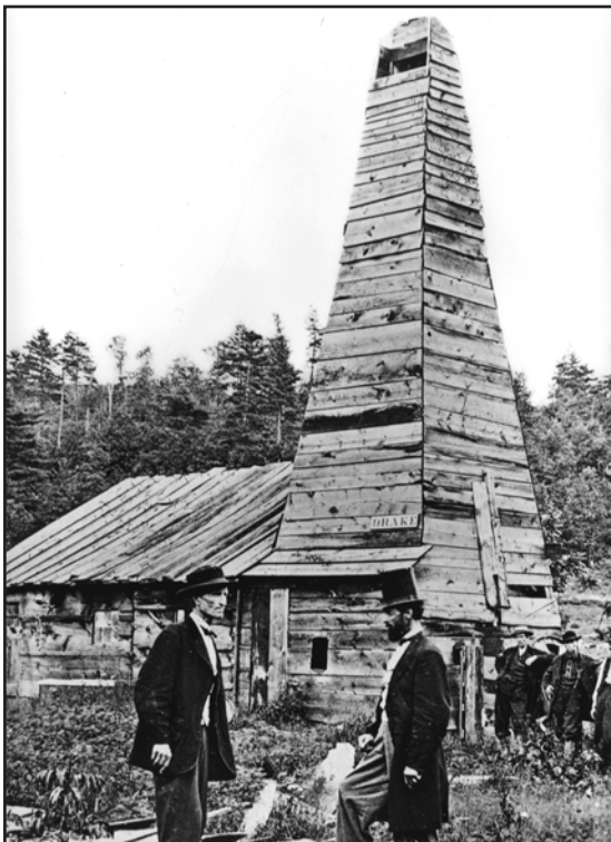
FIGURE 11. The second well drilled by "Colonel" Edwin L. Drake in Titusville, Penn., in 1861. A boiler provided steam to operate a walking beam and churn drill inside in the shack (see end note 41). A pulley mounted at the top of the derrick helped to raise and lower the drilling tools and iron pipe into the hole. This famous photograph shows a bearded Drake with a tall hat (lower right) standing next to the thin-faced Peter Wilson, a Titusville druggist. The photo is a reproduction from the John A. Mather Collection, purchased by J. Carl at the Drake Well Memorial Park in Titusville, Pa., May, 1993.
