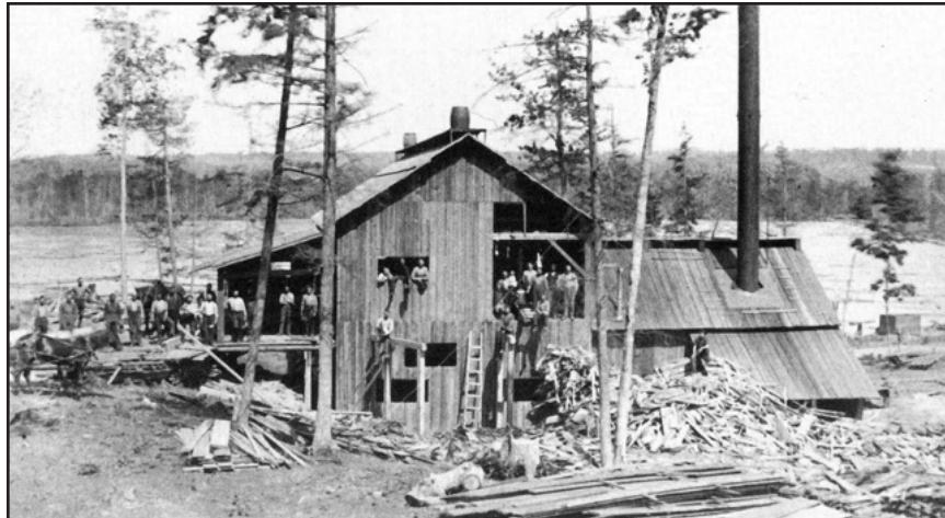
FIGURE 4. Henry Abbey's steam-powered sawmill near the mouth of the Independence River. The sawmill was said to have an annual production of 7,000,000 board-feet of lumber, most of which was shipped on the Black River Canal. The headwaters of this western Adirondack river (behind the sawmill) reach Big Moose settlement and lake north of Eagle Bay. The 1887 photo is from Fynmore and Corwin, 2005, p. 108.
