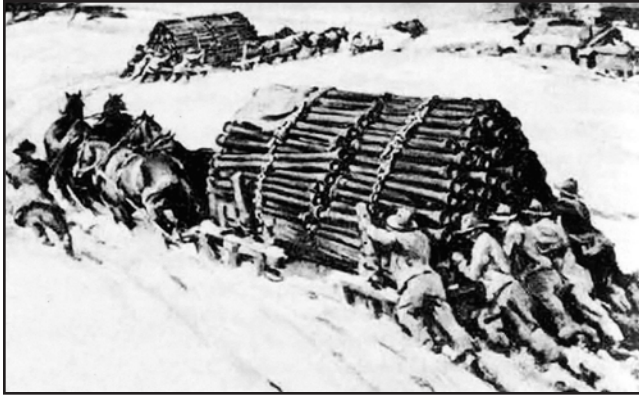
FIGURE 14. Sketch illustrating the construction of the first pipeline across Pennsylvania's Allegheny Plateau by Byron D. Benson's Tide Water Pipe Line Company. Profits from this and other oil related projects would be spent on a railroad and iron mine in the western Adirondacks. Teams of four horses are shown struggling up an incline in winter, hauling sleds loaded with iron pipe. From web site http://www.explorepahistory.com
