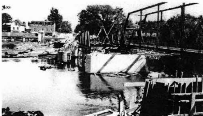
Building the replacement bridge, Rensselaer Falls
