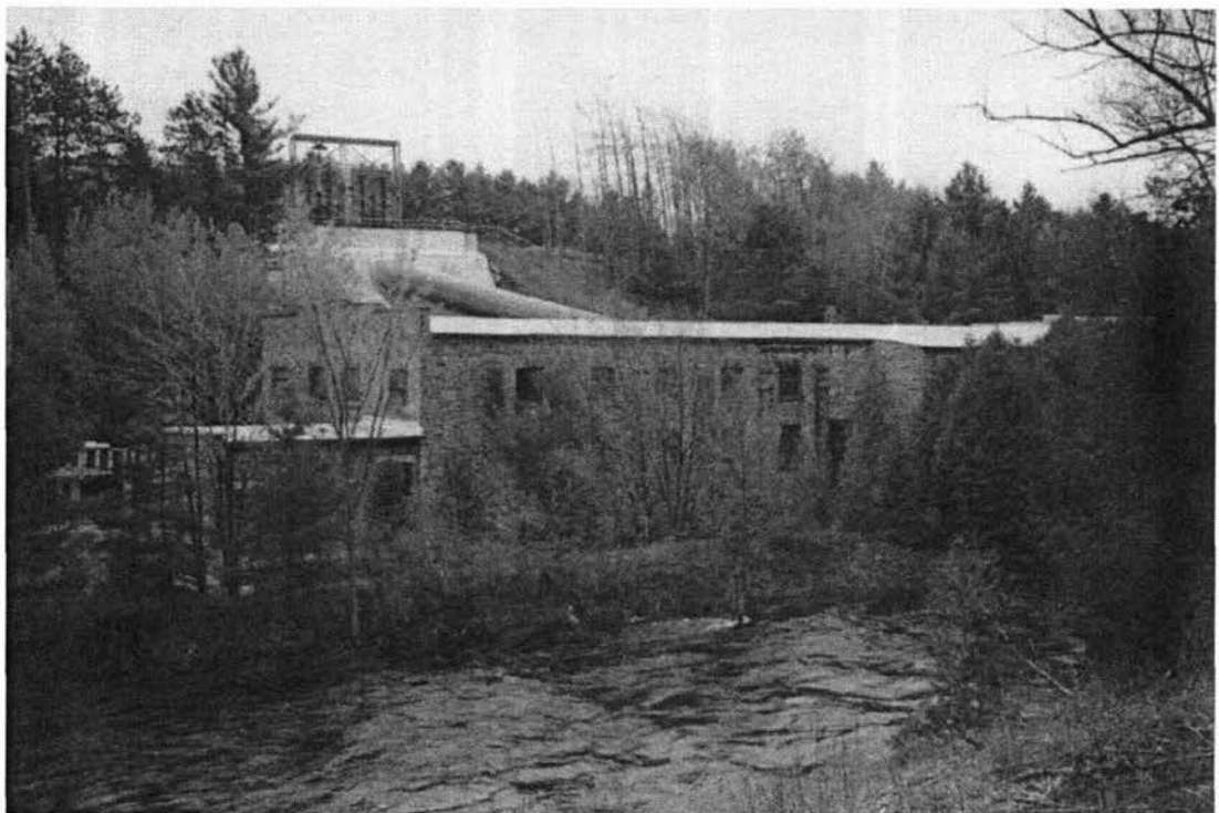
A view of the large Hannawa Falls hydroelectric power plant taken from the west side of the Racquette River, with the canal and penstock behind it.
