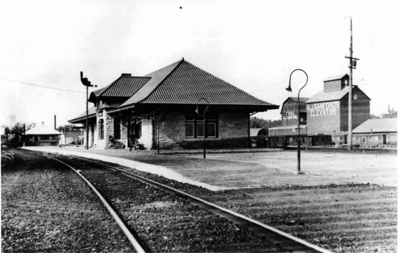
The Potsdam railroad depot in its prime, c. 1914. It was constructed of local red sandstone in a style popular in early 20 th century depots, especially in the Southwest, incorporating broad overhanging eaves, tile roof, and Mission or Craftsman-style details. Photograph from the Potsdam Museum.
