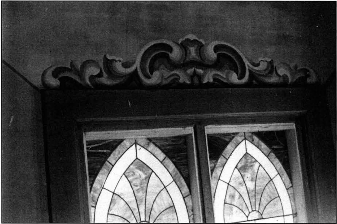
Brick Chapel Church. Stained glass window with painted cap and faux bois wood grain painted window frame. Remnants of Kip's frescoes can be seen in a closed-off choir loft above the entryway. The remainder of his work was painted over and replaced by stenciled designs.
