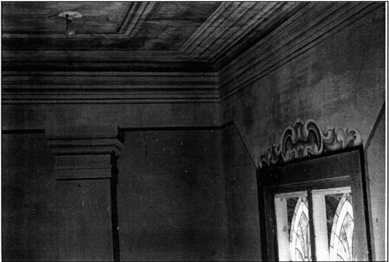
A portion of the frescoing which still remains in the Brick Chapel church probably painted soon after the old church edifice was replaced by a new brick building in 1858. Shown are a painted cornice, ceiling moldings, and the capital of a column motif repeated throughout the interior, and a decorative window cap. It was done in shades of grey accented with black.
