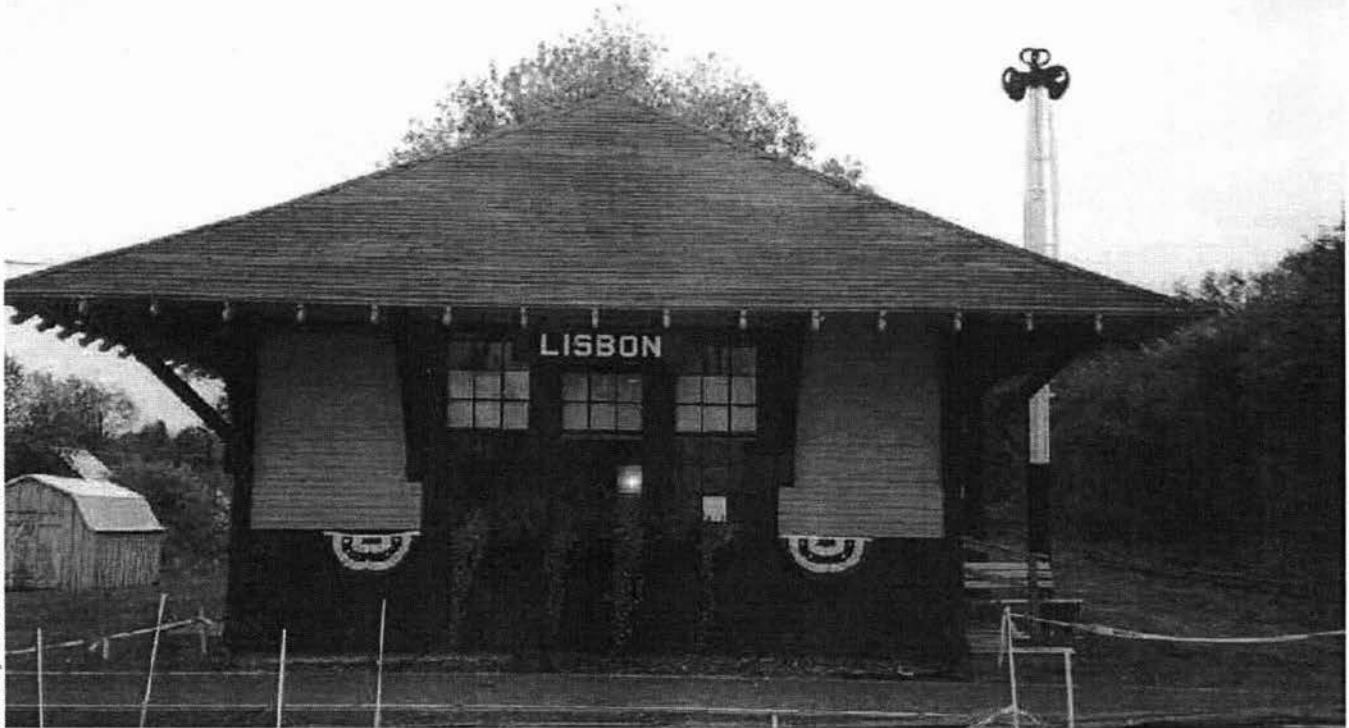
The Lisbon Depot is on the National Register of Historic Places. Historians cite its Bungalow/Craftsman architectural style.
