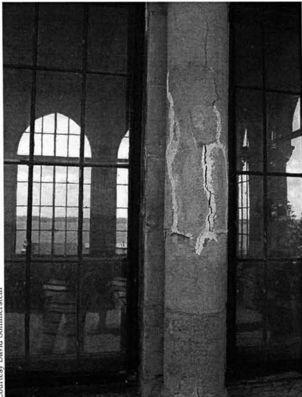
A crumbling concrete support on the porch outside the Breakfast Room testifies to more rehabilitation work that needs to be done.
