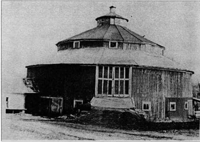
The round barn was built by Charles Flanagan in Southville, Town of Stockholm, in 1906. He styled it after barns he'd seen in the West. It has two silos, one in the center of the barn and one on the outside. The farmer can drive into the barn and pack bales of hay around the inside of the silo.
