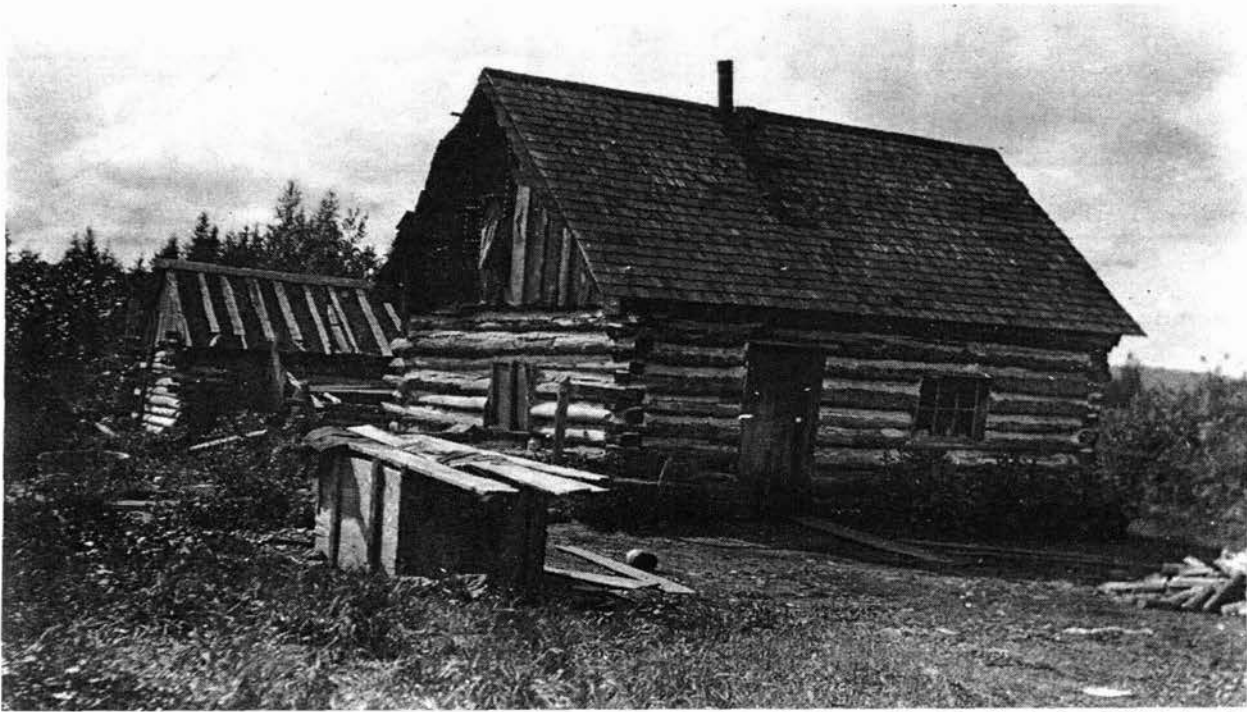
This log cabin located between Sterling Pond and Joe Indian Pond in the Town of Parishville is dated 1903, but is representative of the first dwellings erected by the pioneer settlers, using local materials. Almost all of these small, crude early structures were replaced in time by more permanent frame houses. [1000-1136]
