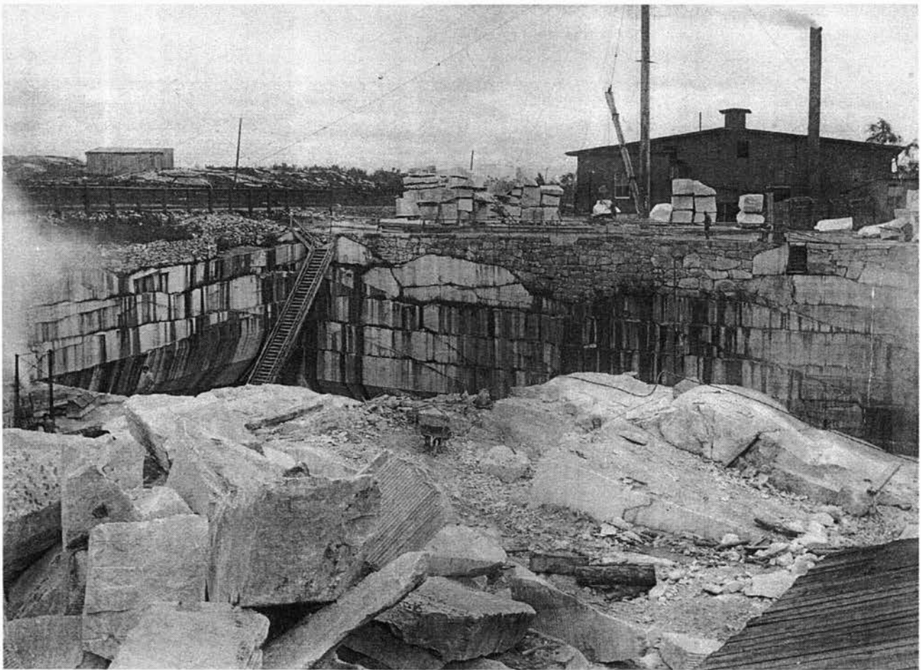
A view of a Gouverneur marble mine owned by St. Lawrence Marble Co. Gouverneur marble is most often seen in late 19 th century buildings. [Potsdam Museum P.151]
