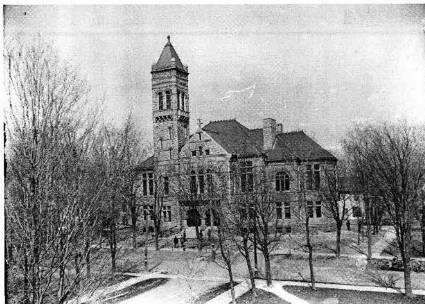
The current courthouse, as it appeared soon after construction in 1896. It was much larger and more elaborate than the first one. The masonry combines use of red Potsdam sandstone with gray Gouverneur marble. [1000-2998]
