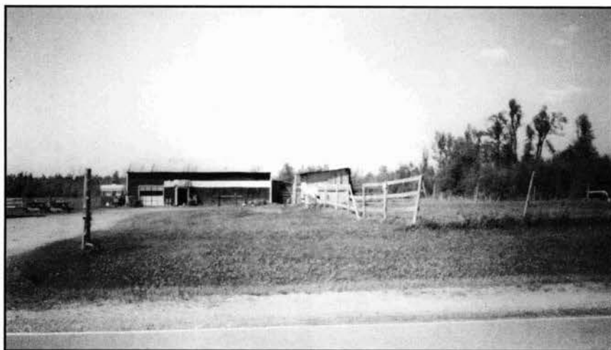
This barn is owned by Beulah Hall, County Route 56. This barn was built in the last few years as a horse barn. She still has a horse and also a goat.
