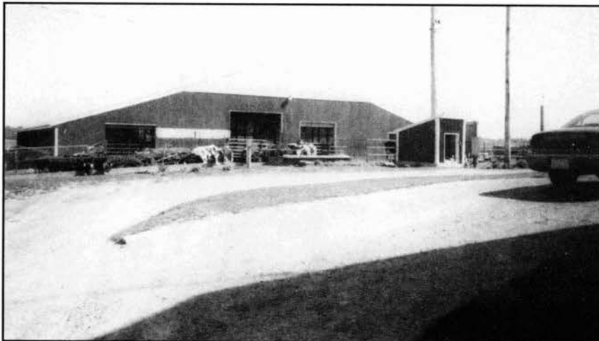
Barn in back of the house for milking cows, built in 1984.
