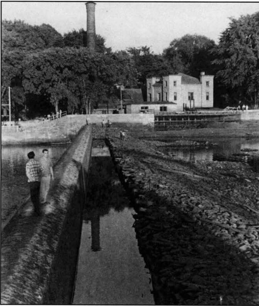
In this picture taken in the early 1960s, Ford's Dam can be seen behind the new concrete dam built in 1910.
