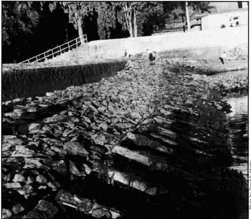
Here is a clear view of the water face of Ford's Dam. Some of the timbers and planks from which the deck was constructed can be seen. The deck allowed ice and debris to slide smoothly over the dam without causing a jam.
