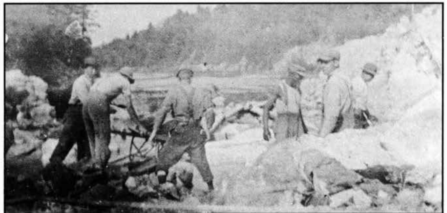
Removing rocks from the channel in the river.
