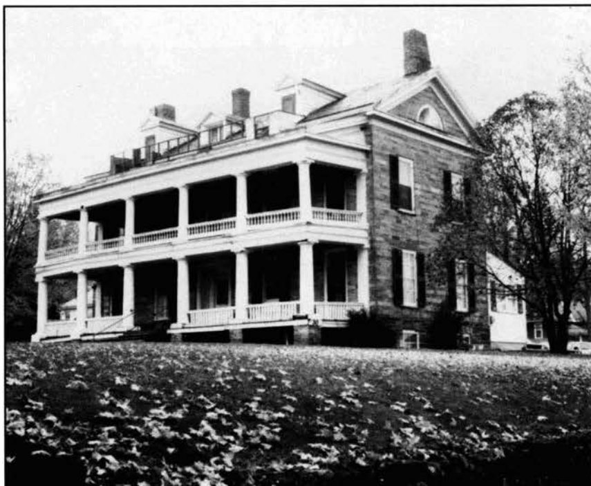
The 1836 David Clarkson mansion, later known as the General Merritt house. The Clarksons' influence in sandstone architecture is evident in that several stone houses in the Greek Revival style were constructed soon after this one.
