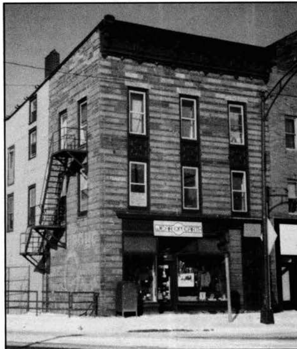
The former Hopkins Tannery at 1 Market St. is a well-preserved example of slab and binder masonry in a commercial structure.
