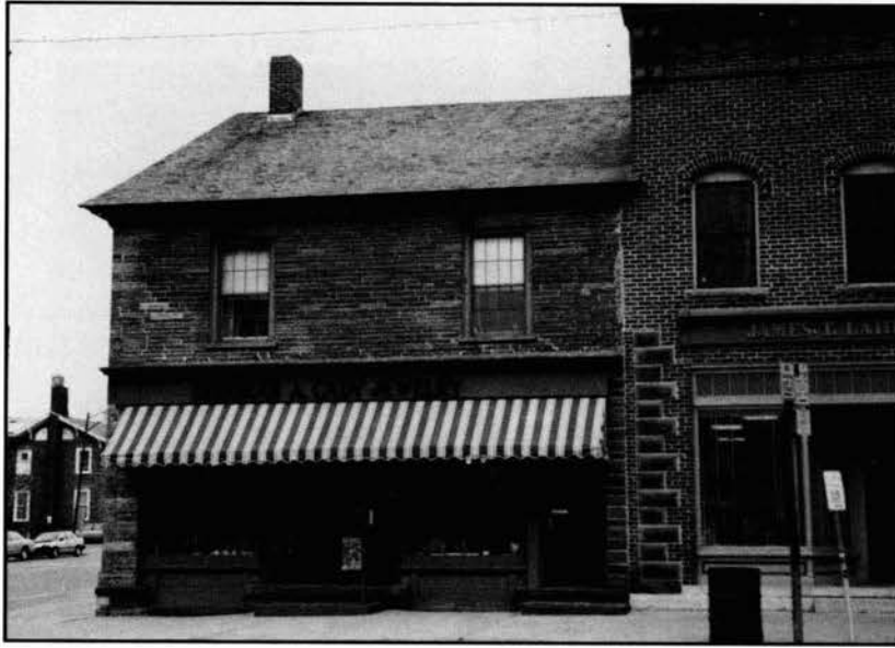
Potsdam's first sandstone building, at 30 Market Street. Note the small size of the stones.
