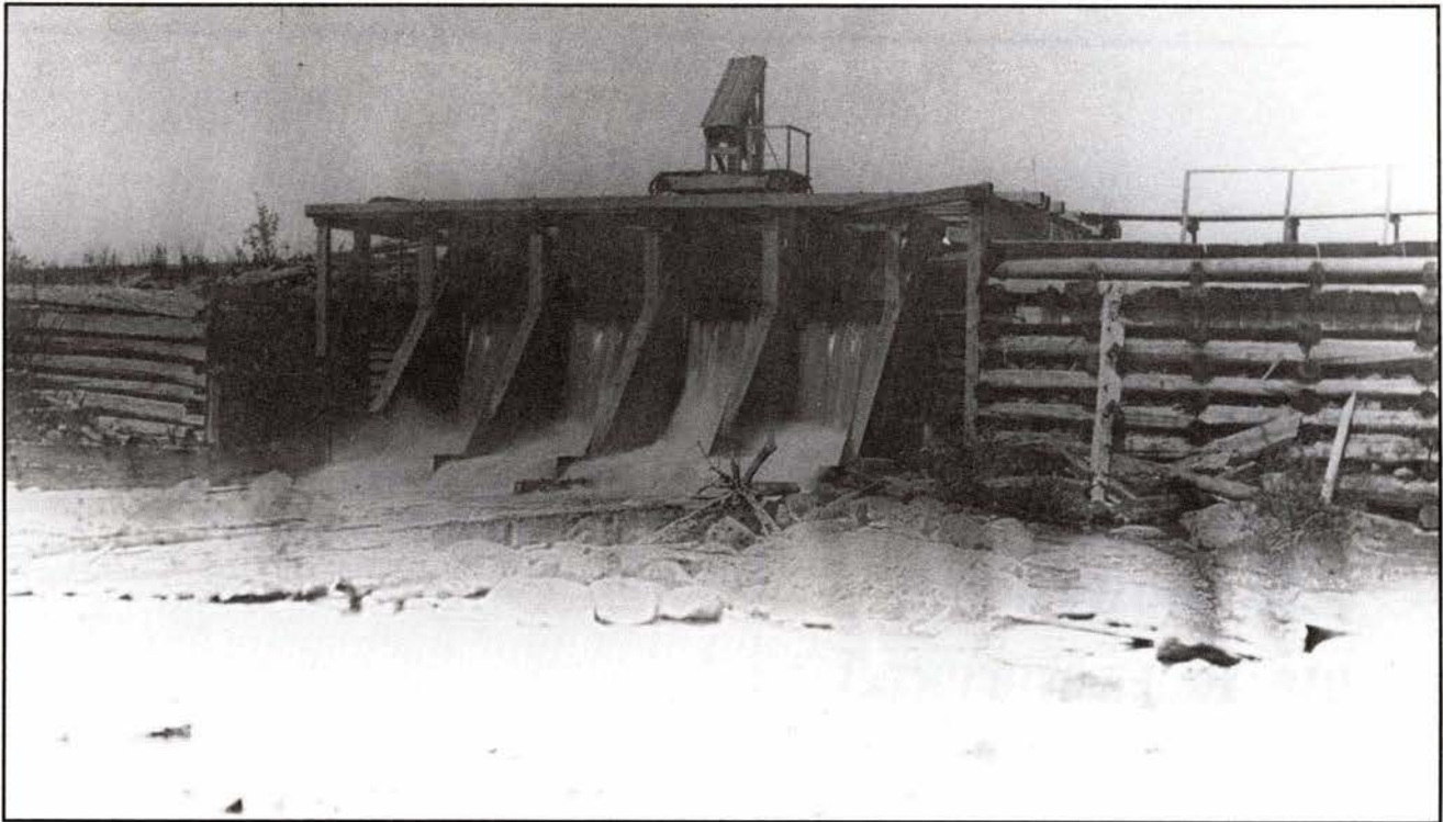
The original Cranberry Lake Dam
