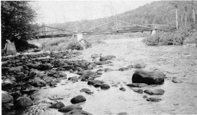
The Jordan Bridge, circa 1934 (Photo courtesy of Bob Stoddart)
