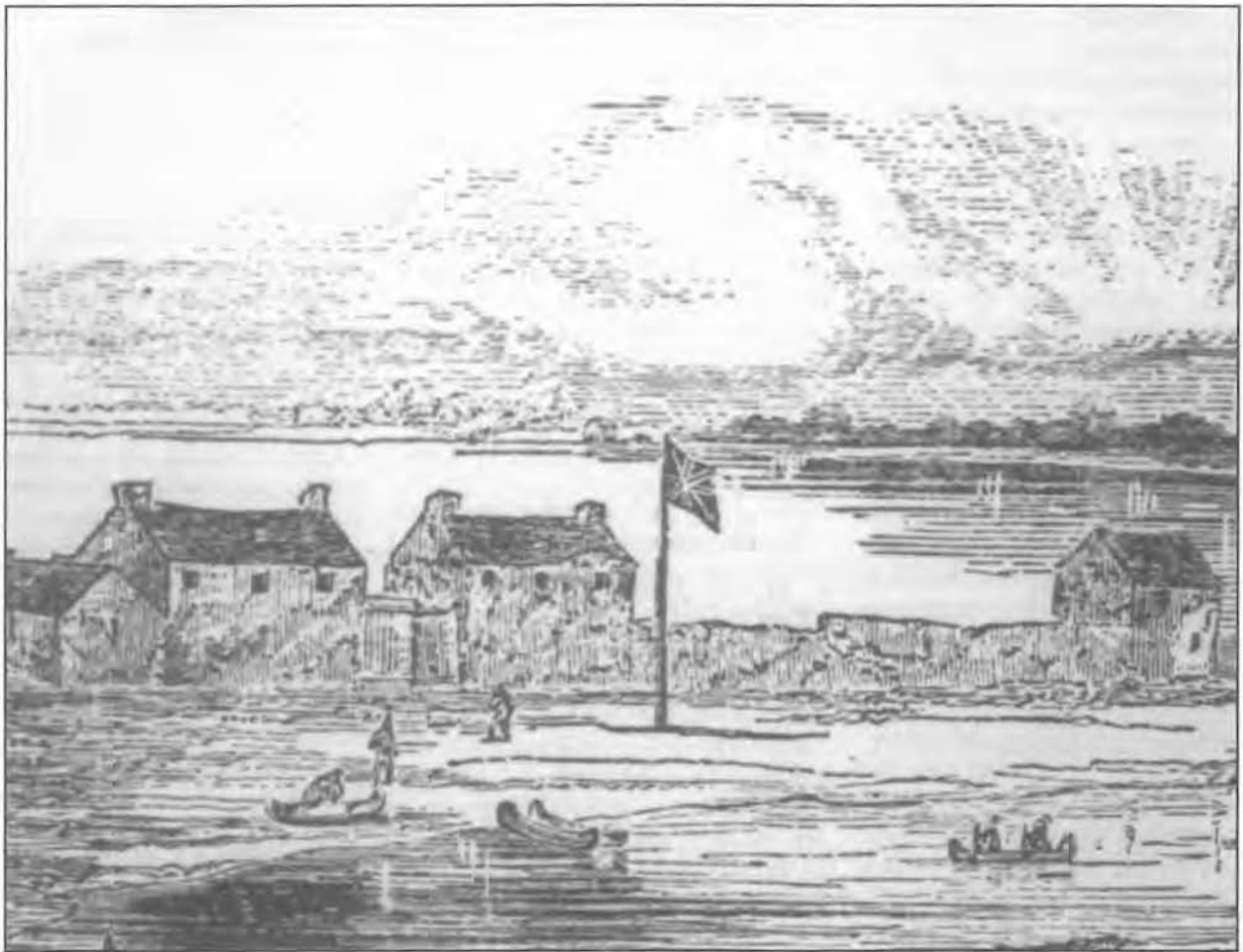
Fig. 3: The Hangar (Store House), Small House (Later, the Bastion to the Fort), Stone Redoubt, Barn, and Oven Built by Father Picquet in 1749 (Photo after Rt. Rev. P. S. Garand, The History of the City of Ogdensburg)
