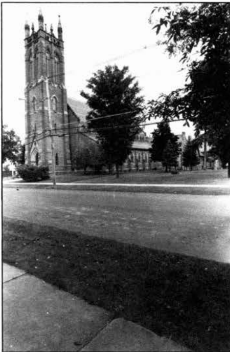
Fig. 5: Ogdensburg. Second Church of St. John the Evangelist. 1870. Architect: Emlen T. Littell. (Photo by Adam Markowitz)
