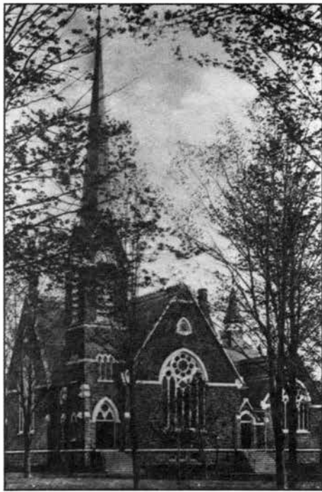
Fig. 7: Canton. Second Presbyterian Church. 1876. Architect: James P. Johnston. (Courtesy of St. Lawrence County Historical Association Archives)
