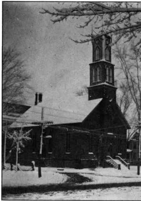
Fig. 8: Potsdam. First Methodist Church. 1860. Architect Unknown. (Photo courtesy of Douglas Arquette)
