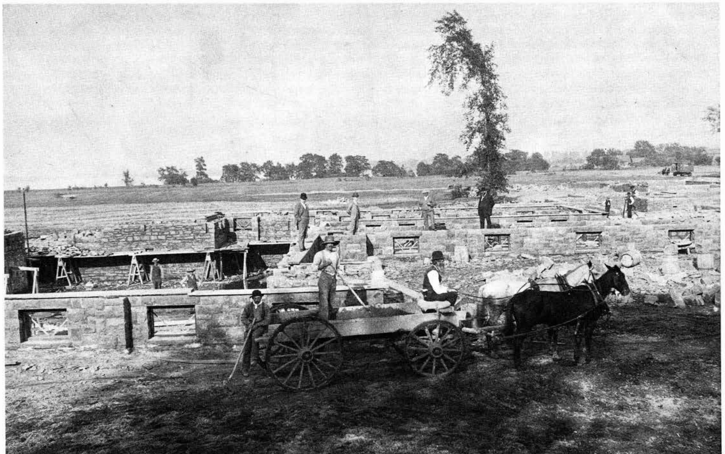
Using Gouverneur light gray limestone and Potsdam red sandstone construction of Center Building began in 1888.
