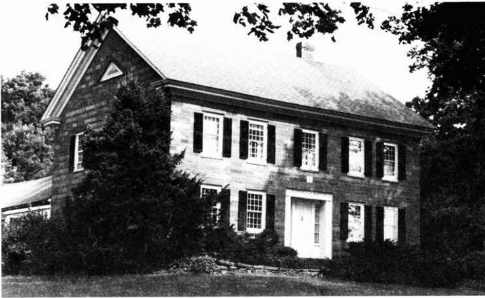
The Omohundro house, Hannawa Falls, formerly the Gardner Cox home. (Photo by Marian O'Keefe, SLCHA Archives)
