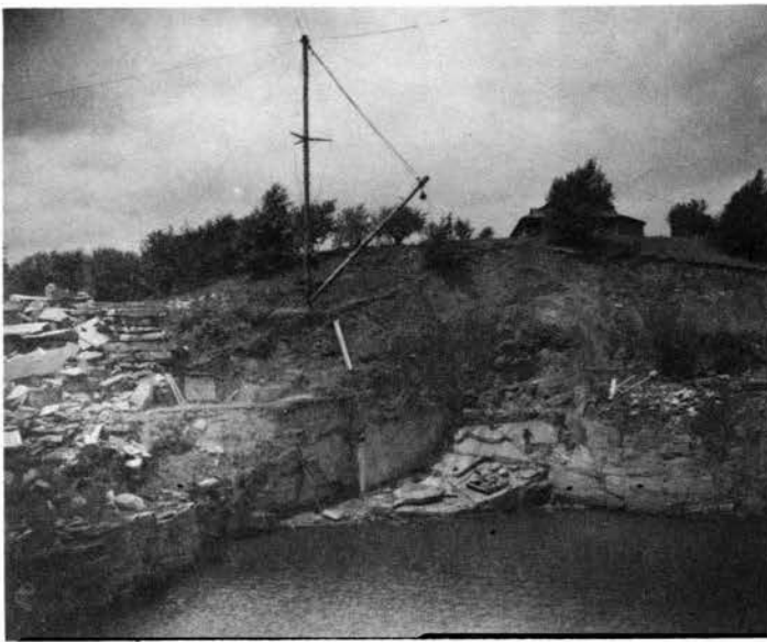
A worksite along the Racquette River. (Courtesy of the St. Lawrence University Archives)
