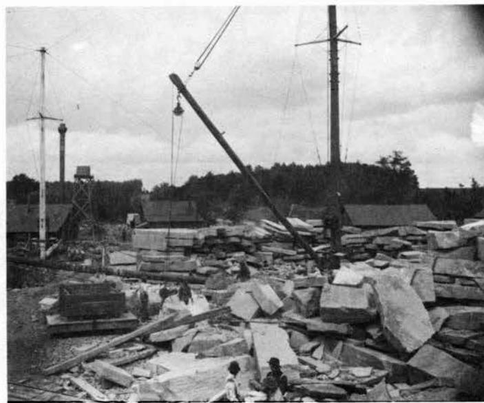
Moving and stacking slabs of Potsdam sandstone. (Courtesy of the St. Lawrence University Archives)
