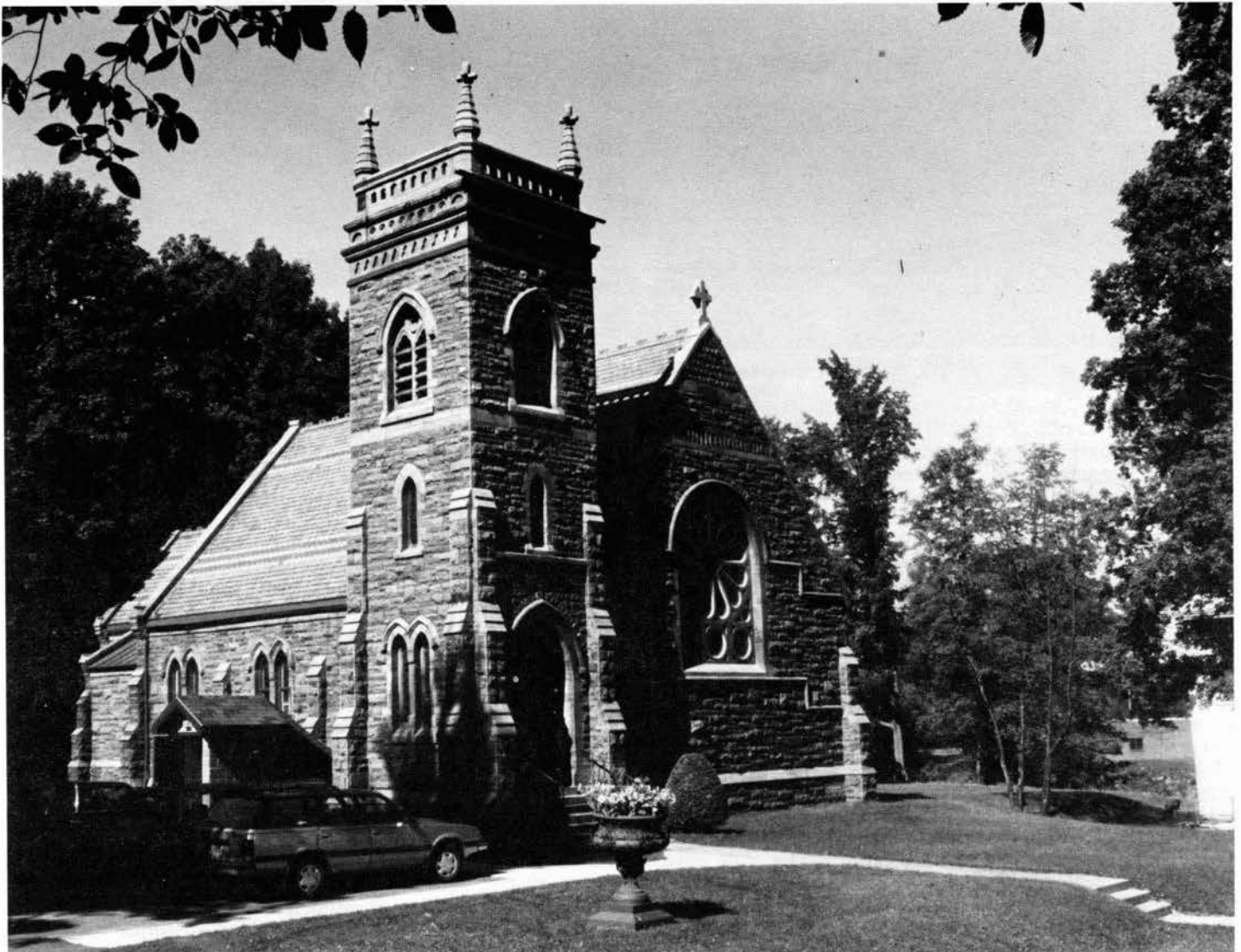
Fig. 7: Zion Church, Colton. Exterior View from Northwest. 1990. (Courtesy of Adam Markowitz)
