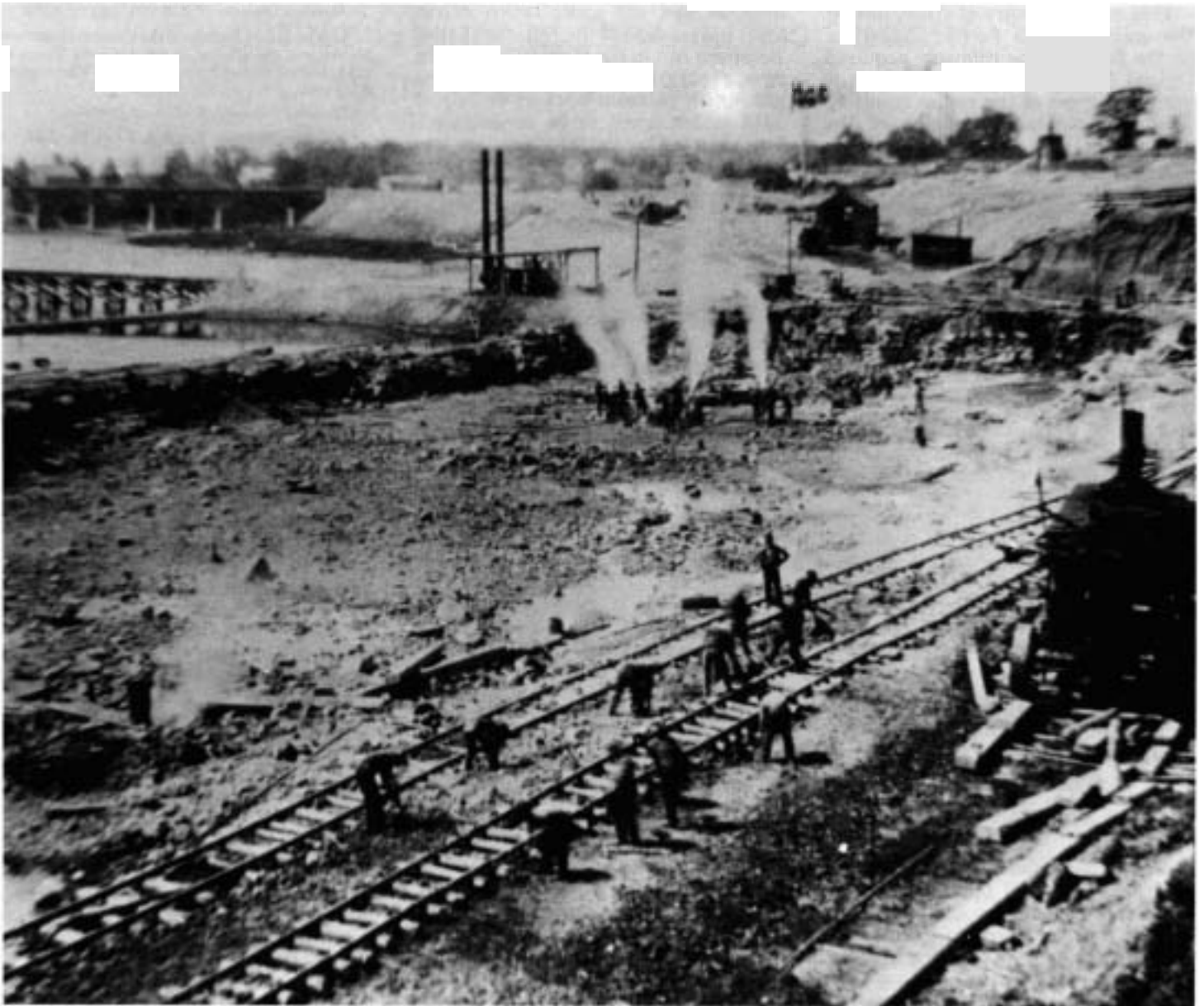
Power Canal Construction, Massena, NY, 1898. (Archives, SLCHA)
