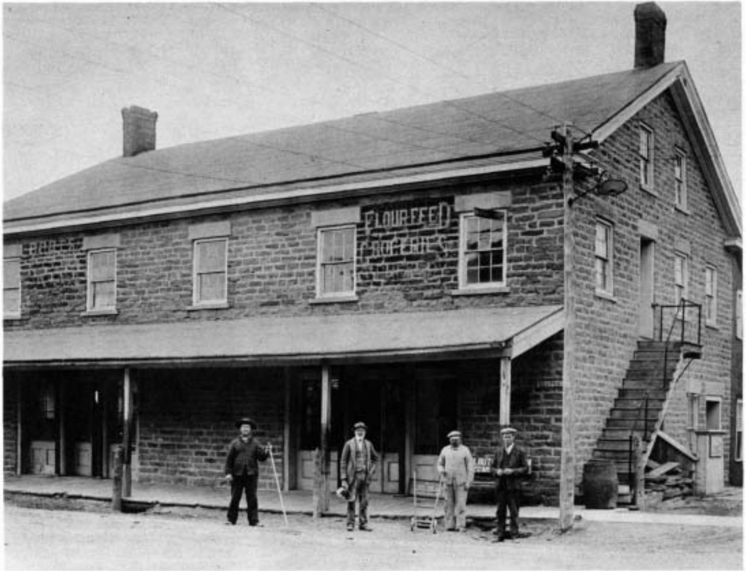
Nathan Ford Giffin erected in 1853 this stone building at the northwest end of the bridge on State Street. He was a dealer in boots, groceries, harnesses and also had a tannery. In 1887 George C. McFadden and his father-in-law, Charles P. Anderson, formed a partnership and purchased the Giffin store, and established a grist mill and feed store. The business was operated until 1916 when the illness of Mr. McFadden forced him to sell the business to Henry G. Mayne and son. In 1943 the building was purchased by Stanley and Alice Richardson. Dan S. Giffin's law office is believed to have been in the second floor right hand corner where the Notary Public sign can be seen. This picture was taken after 1906, because that year electricity came to Heuvelton. The men are identified as John Crawford, Jr., Charles P. Anderson, Harlan Smithers, and William Smith. (Photograph courtesy of the Heuvelton Free Library)
