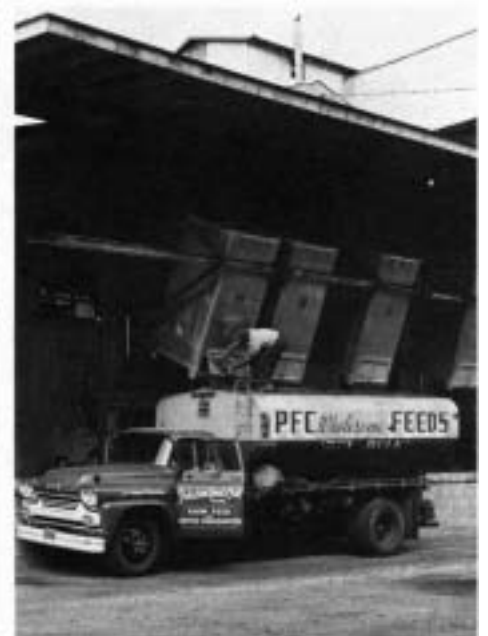
Signs of modernity in the new mill: Left, grain from a mixer fills a tote bin; center, tote bin is "toted" to rack; right, truck loads from tote bin. (Photographs courtesy of Dorothy Jones Gordanier)
