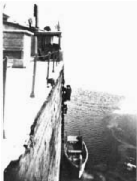
D. D. Hill climbs Jacob's ladder on the Compton to make a winter inspection in 1918. (Photograph courtesy of Ralph E. Hill)
