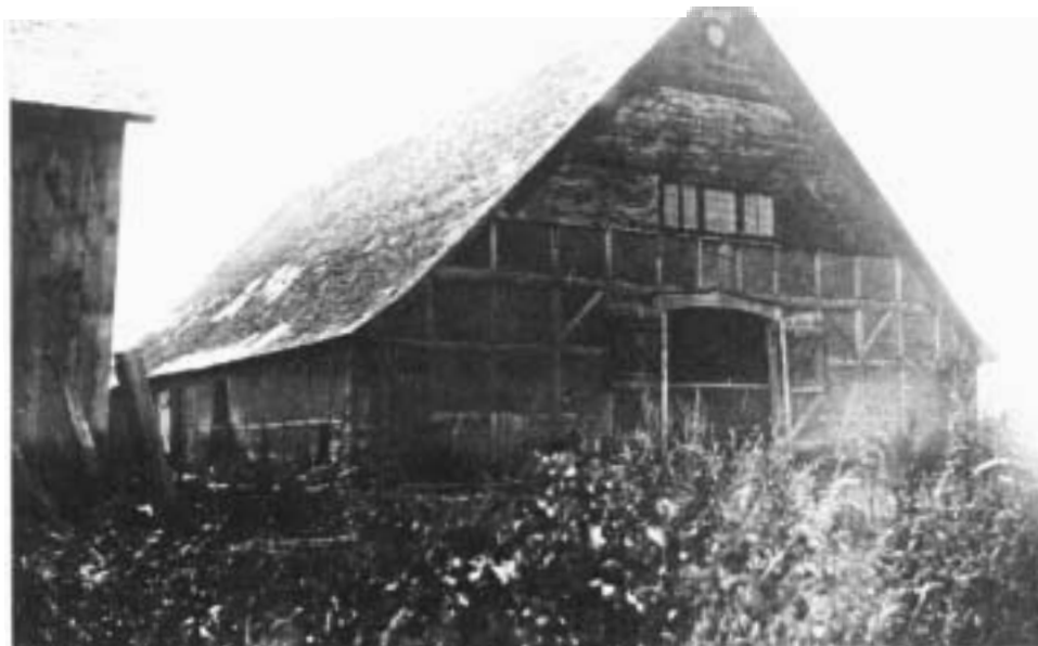
Fig. 10: Early photograph of the east end of the barn, showing the brick infill of the timber wall structure. (Photograph, courtesy of Mary C. Burroughs and Virginia Ward Duffy McLoughlin, now in the St. Lawrence County Historical Association archives)
