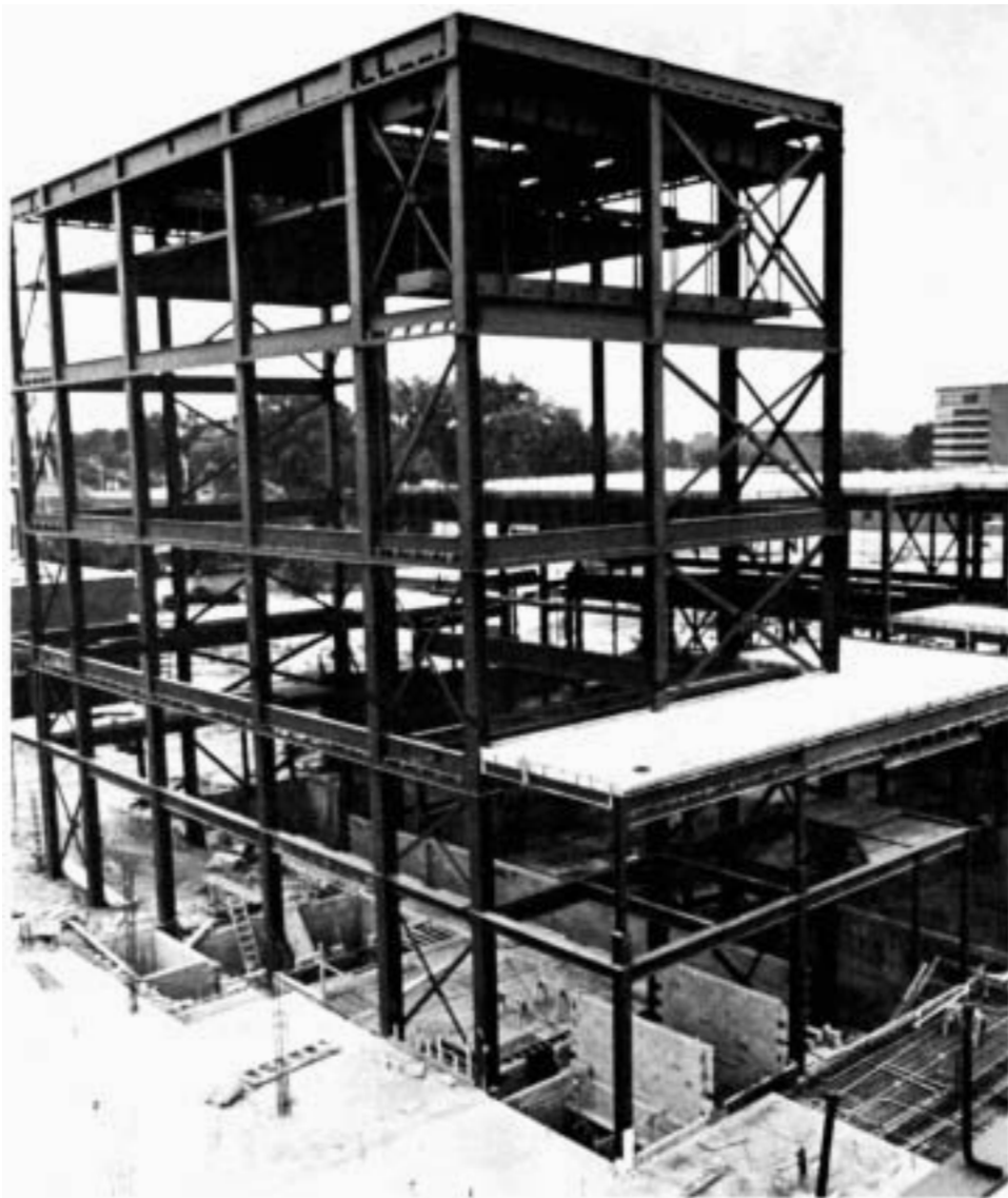
The new Crane complex under construction. (Photograph by Sal Cania)
