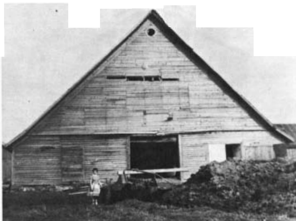
Fig. 11: West end of the barn in 1956. (Photograph courtesy of the St. Lawrence County Historical Association archives)
