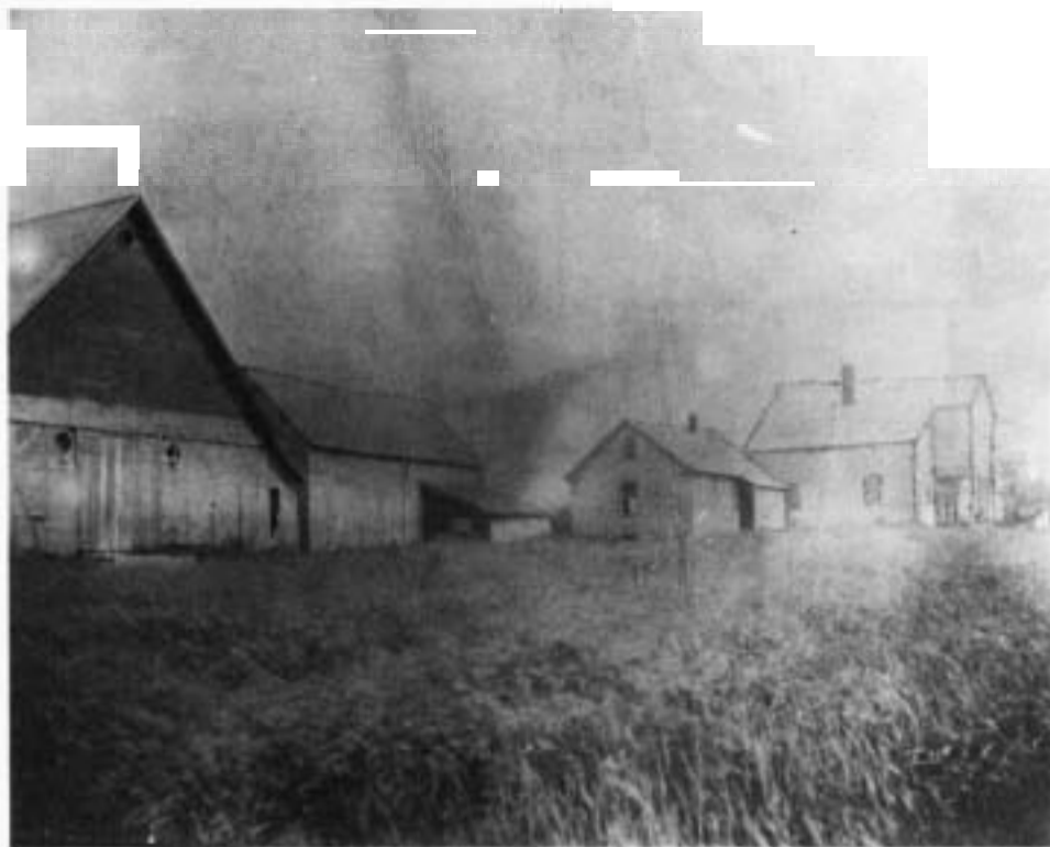
Fig. 5: The barn and the house, seen from the northwest. Retouched photograph. (Photograph, courtesy of Mary C. Burroughs and Virginia Ward Duffy McLoughlin, now in the St. Lawrence County Historical Association archives)
