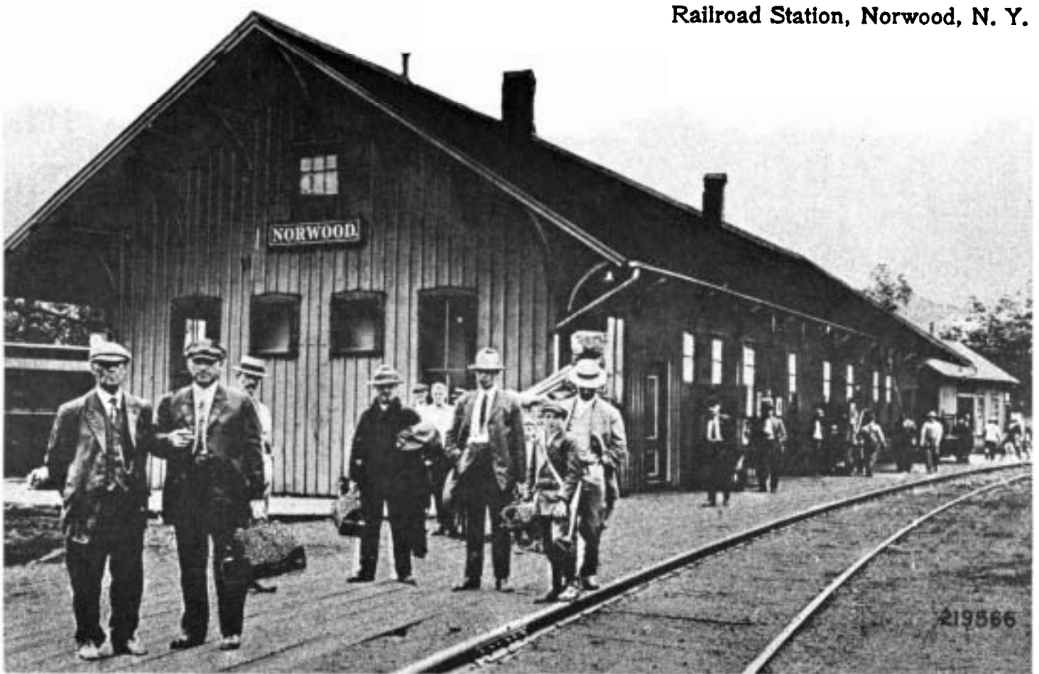
Norwood station, the busiest in the county, with thirteen departures daily in the summer of 1945. The New York Central track is in the foreground; the Rutland's track is on the other side of the station. The Norwood and St. Lawrence Railroad also operated from this station. (Photograph courtesy of the St. Lawrence County Historical Association Archives)
