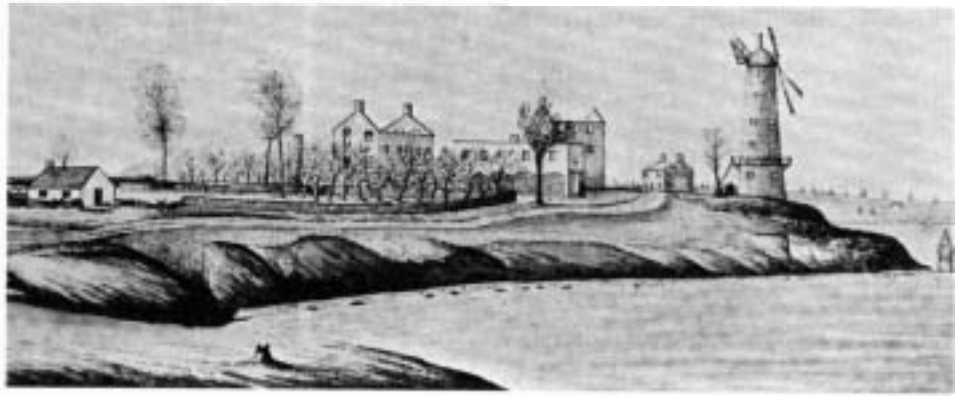
H.F. Ainsley's April 1839 sketch of the Prescott Windmill and surrounding buildings. (Picture courtesy of the St. Lawrence County Historical Association Archives)
