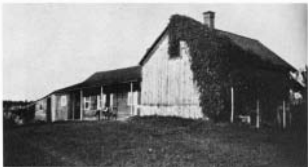
The Shipman house on Wilson Road in Pierrepont, built by Albert Shipman between 1865 and 1868. The front was made of logs and later boarded over.
