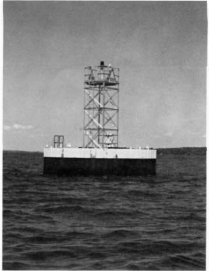
Fixed marker Number 160 installed off Crossover Island in 1980. (Photo by John Ranlett)
