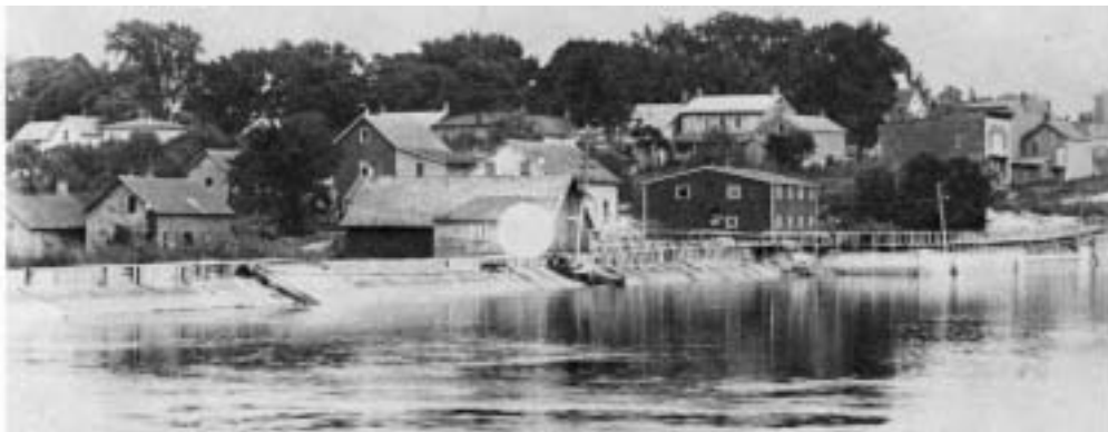
Dam and businesses along Canal Street in Waddington, now under water. Lower end of Main Street. Building on shore at right was moved to Maiden Lane and is now used as Gib's Restaurant. (Photo courtesy of Pauline Tedford, Town of Waddington Historian)
