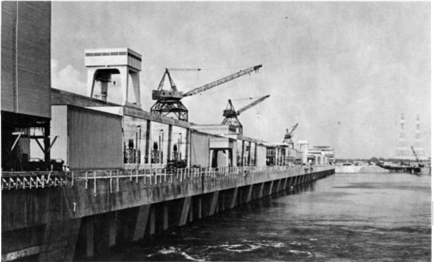
General view of the downstream face of the St. Lawrence Power Dam. (Photo courtesy of the Dumas family of Massena)
