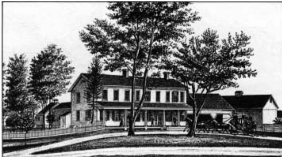
The Ira French tavern and homstead, Town of Potsdam, is a good example of an early New England Georgian structure.
