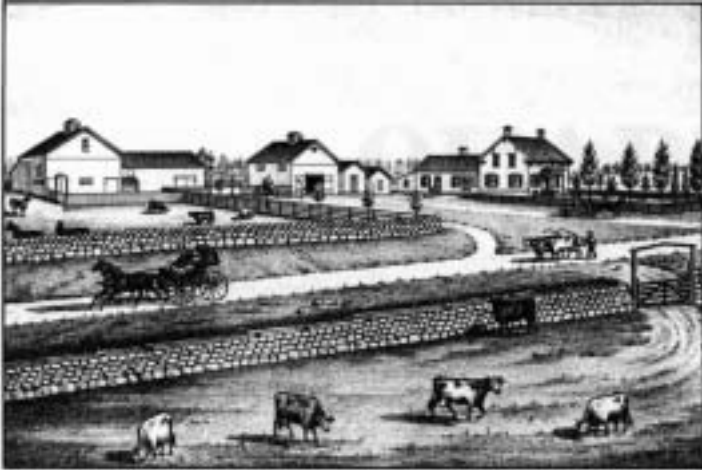
Note the diamond window in the central barn's gable end, and the cupola vents on both barns. Contrast this with the absolute plainness of the barns in the slightly more traditional Crouch homestead.
