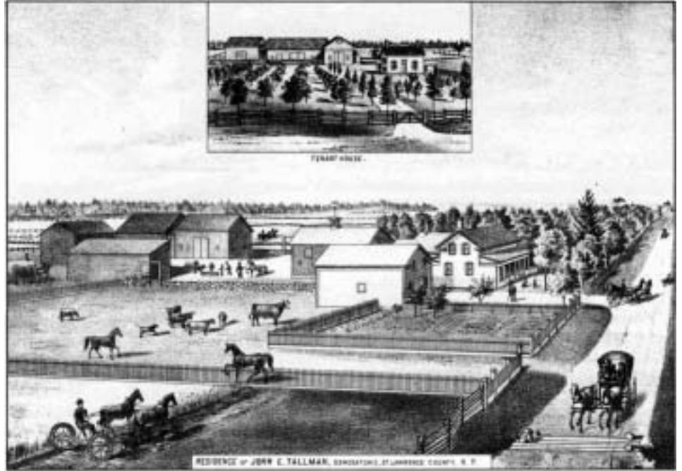
On the Tallman farm English side opening barns were arranged around a courtyard or barnyard. Note that the scale of farming in the 19th century made the use of several small barns more effective than resort to one or two very large barns. Note also the absence of silos from all the Evert engravings in 1878.
