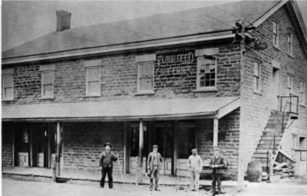
Nathan Ford Giffin erected in 1853 this stone building at the northwest end of the bridge on State Street. He was a dealer in boots, shoes, groceries, harnesses and also had a tannery. In 1887 George C. McFadden and his father-in-law, Charles P. Anderson formed a partnership and purchased the Giffin store, and established a grist mill and feed store. The business was operated until 1916 when the illness of Mr. McFadden forced him to sell the business to Henry G. Mayne and son. In 1943 the building was purchased by the present owners, Stanley and Alice Richardson. This picture taken after 1906, for that year electricity came to Hewelton. In upper left can be seen word "Boots" and on upper right "Flour, Feed, Groceries" advertising the business when owned by Giffin. The men are identified as John Crawford, Jr., Charles P. Anderson, Harlan Smithers and William Smith.
