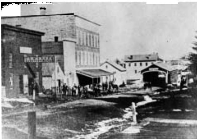
This picture taken between 1870 and 1875. The last covered bridge at Heuvelton built to replace the one carried away by the flood waters April 18, 1862. On left side of street J.D. McBroom, carriage maker. The J. Best Store next to large three story store building built in 1858 by John Pickens, Sr.
