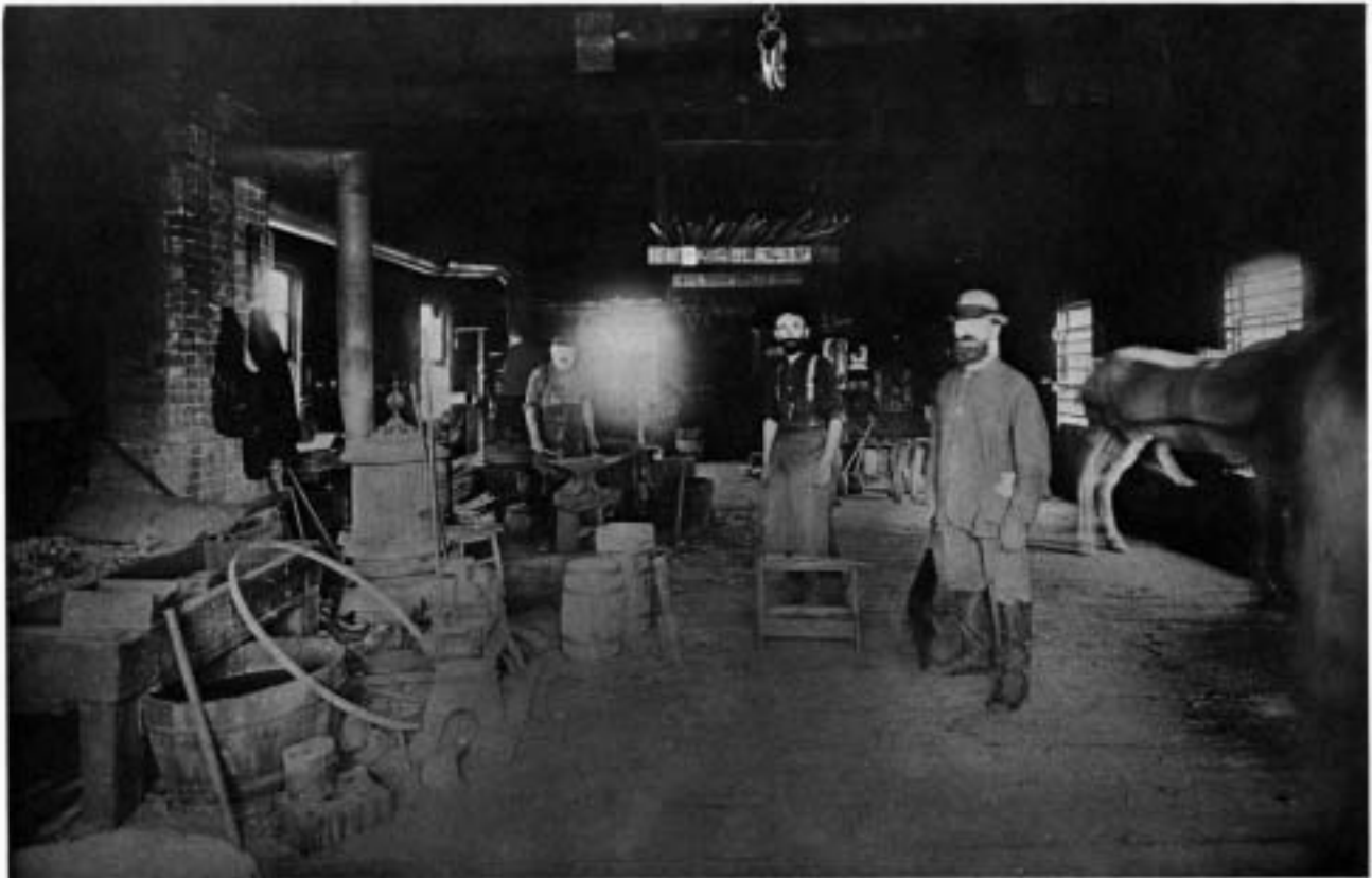
Interior of a blacksmith shop in Heuvelton. In 1900 there were four blacksmith shops in Heuvelton.
