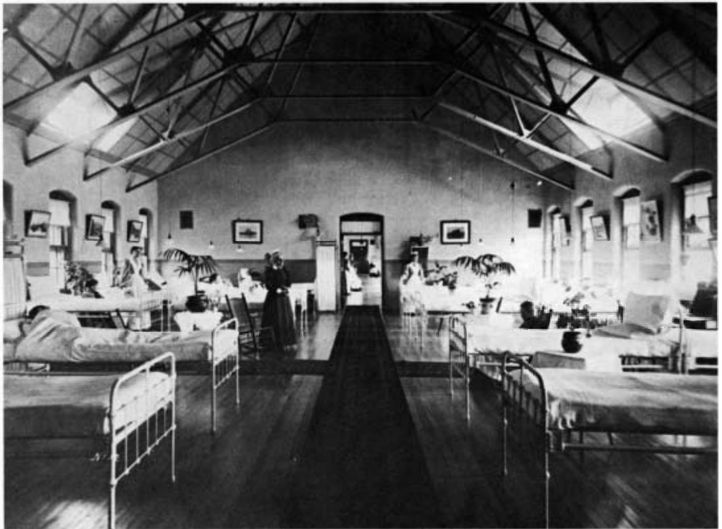
Letchworth day room. Note the open truss ceiling. One of the tenets favored by Dr. Wise was that each patient was to have 600 cubic feet of space. One way to do this without increasing the building dimensions was to build up—hence the high open ceilings. (Courtesy St. Lawrence Psychiatric Center)
