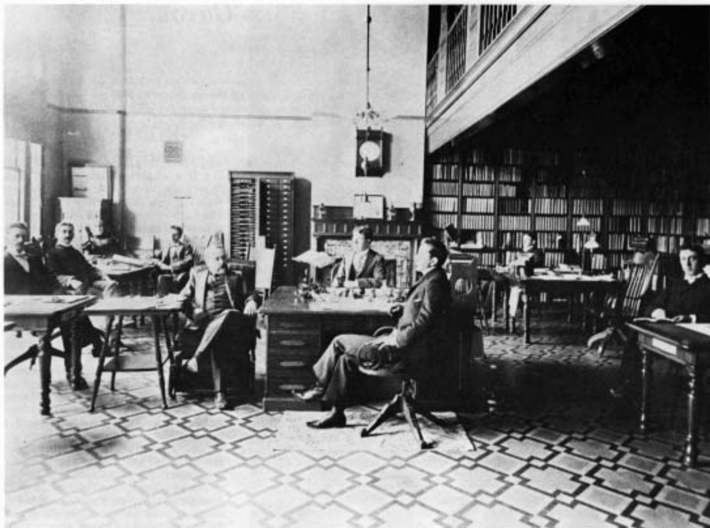
Medical library in building directly behind the administrative offices. Note the encaustic tile floor, which remains to the present day, and the balcony of white oak, which has been removed. (Courtesy St. Lawrence Psychiatric Center)
