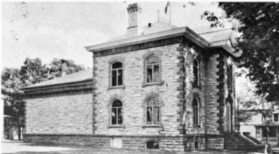
St. Lawrence County Clerk's Office, now the Surrogate Court building. (Photo by R.B. Dezell, Canton, courtesy of SLCHA Archives)
