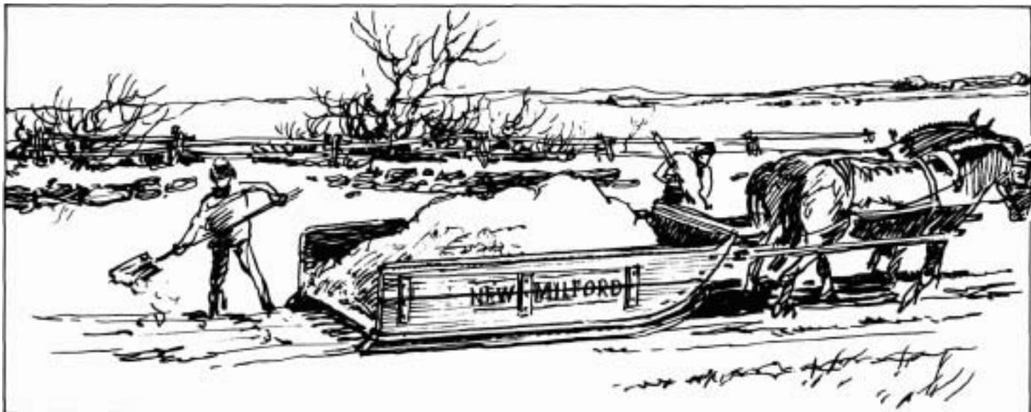
Sketch of men "snow paving" or leveling out the snow cover of rural highways to make for better sleighing. (Courtesy of Eric Sloane's American Yesterday , Wilfred Fauk, Inc.)
