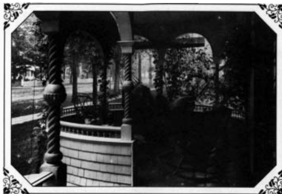
Porch of George Malby House, Ogdensburg.
