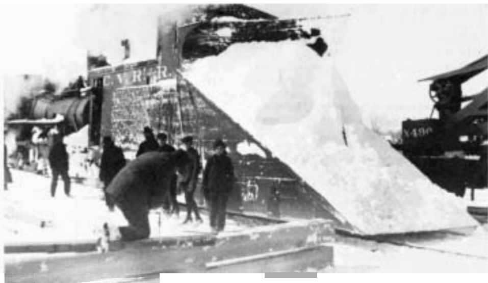
Snow plow used on Ogdensburg and Champlain Valley branch of Rutland Railroad (formerly the Northern) at Malone. (Photo on glass plate negative by Guy Dewey, courtesy of Robideau Studios and the Franklin County Historical and Museum Society)
