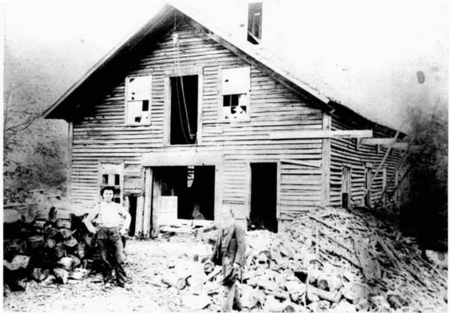
The sawmill and shingle mill of the E.E. and C.C. Green Company which was constructed in 1894. The mill had an up-and-down (vertical) saw powered by water. This building burned in 1913. (Photo courtesy of the author)
