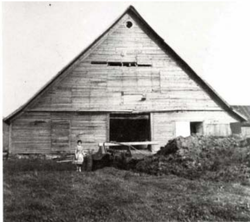
A view of the back of the old Parish sheep barn near Parishville, taken in 1955. The barn was built in 1813 and burned in 1959. (Photo courtesy of History Center Archives)
