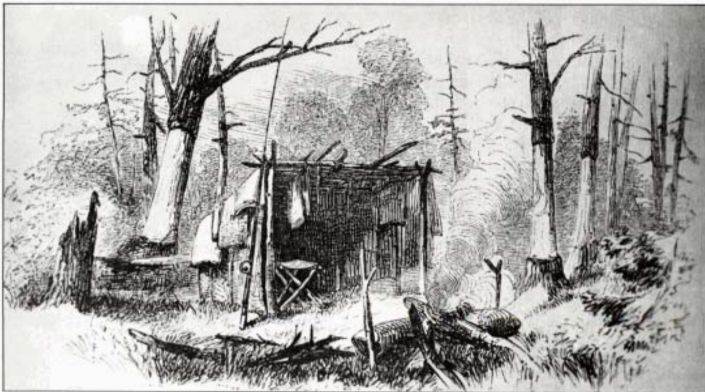
Hunter's shanty similar to those that sheltered Irving's party on August 14 and 15, 1803. Some had siding of bark, others of logs. Roofs were of bark or boughs. Shanties also provided temporary housing for pioneers pending the building of log cabins. Daniel Boone left a trail of them on his way to Kentucky, and Abe Lincoln's family lived in a three-sided shanty their first year in Indiana. Shanties were the ancestors of the Adirondack lean-to of today. (From Harper's Magazine, 1859)
