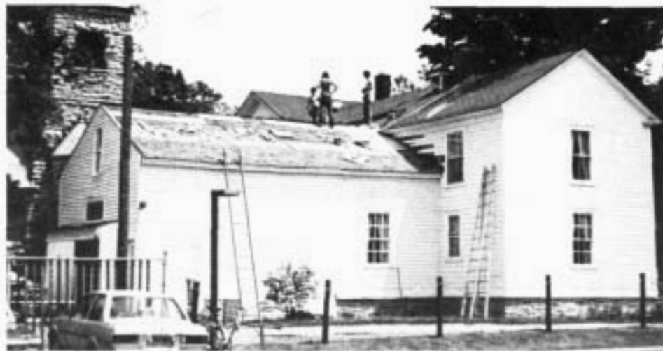
Workmen restoring cedar shingle roof on Silas Wright House.
