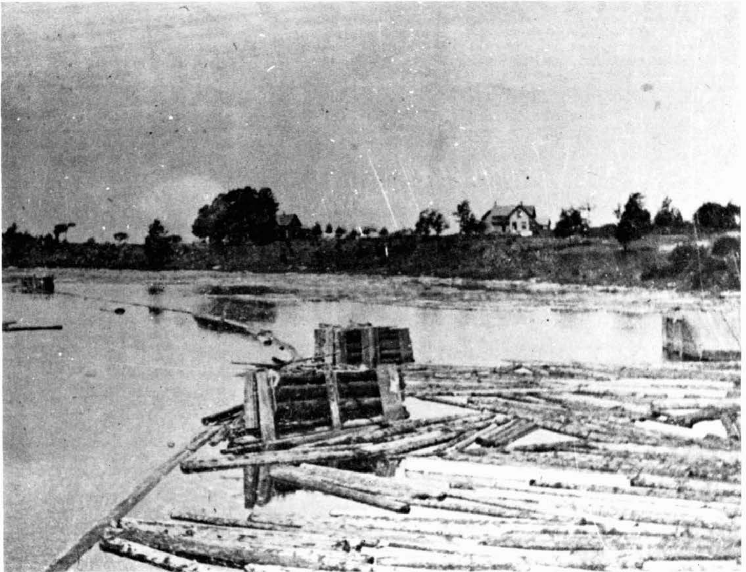
A logging boom on the Grass River. The cribs built of logs and stones kept the booms from drifting to shore. (Photo courtesy of the author, from the History Center Archives)
