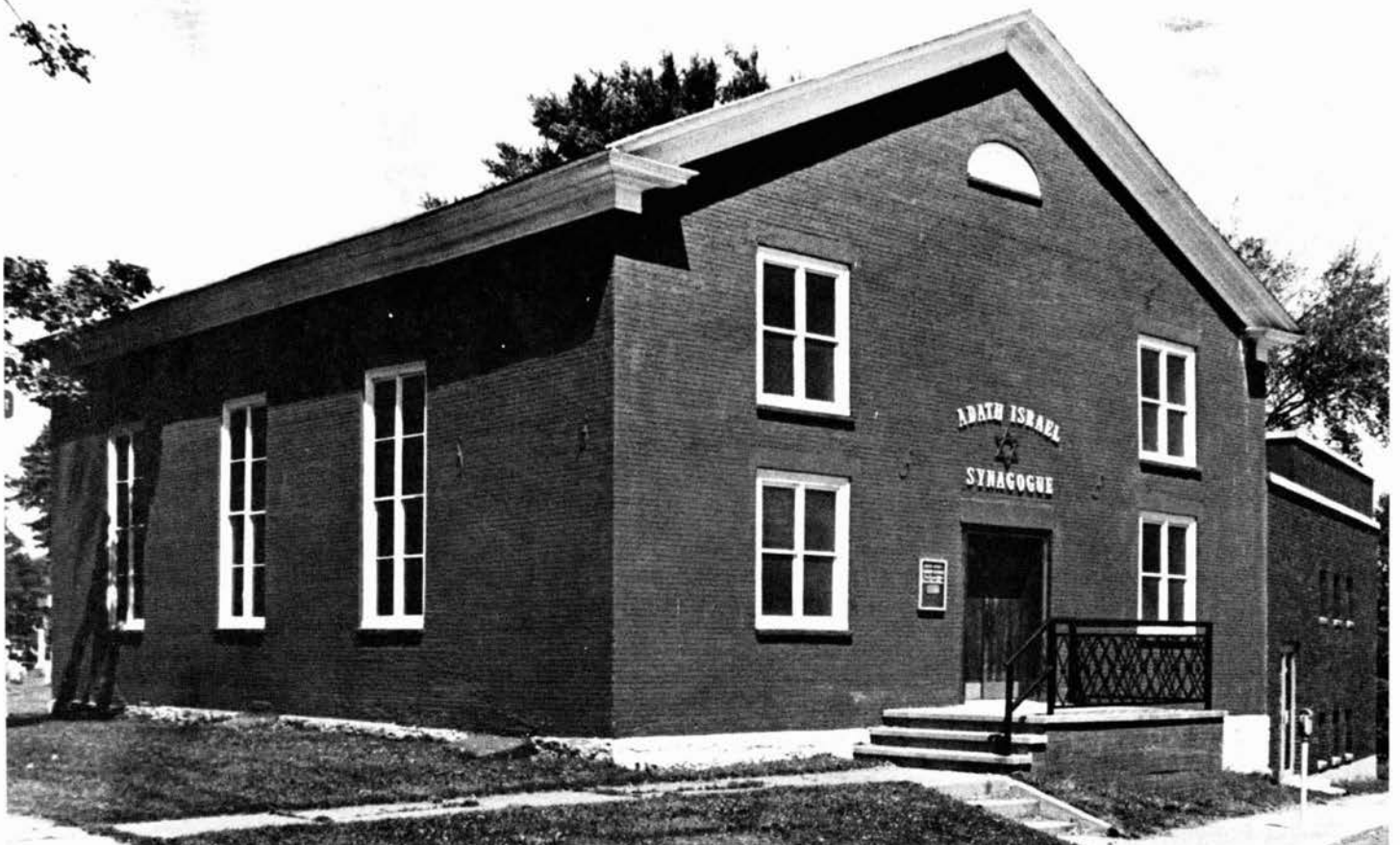
Adath Israel Synagogue, on Church Street in Massena, was built in 1844 as a Congregational Church of local red brick from a kiln on Center Street. The Jewish congregation bought the building in 1921, removed the steeple, added a community center and a new decorative entrance.
