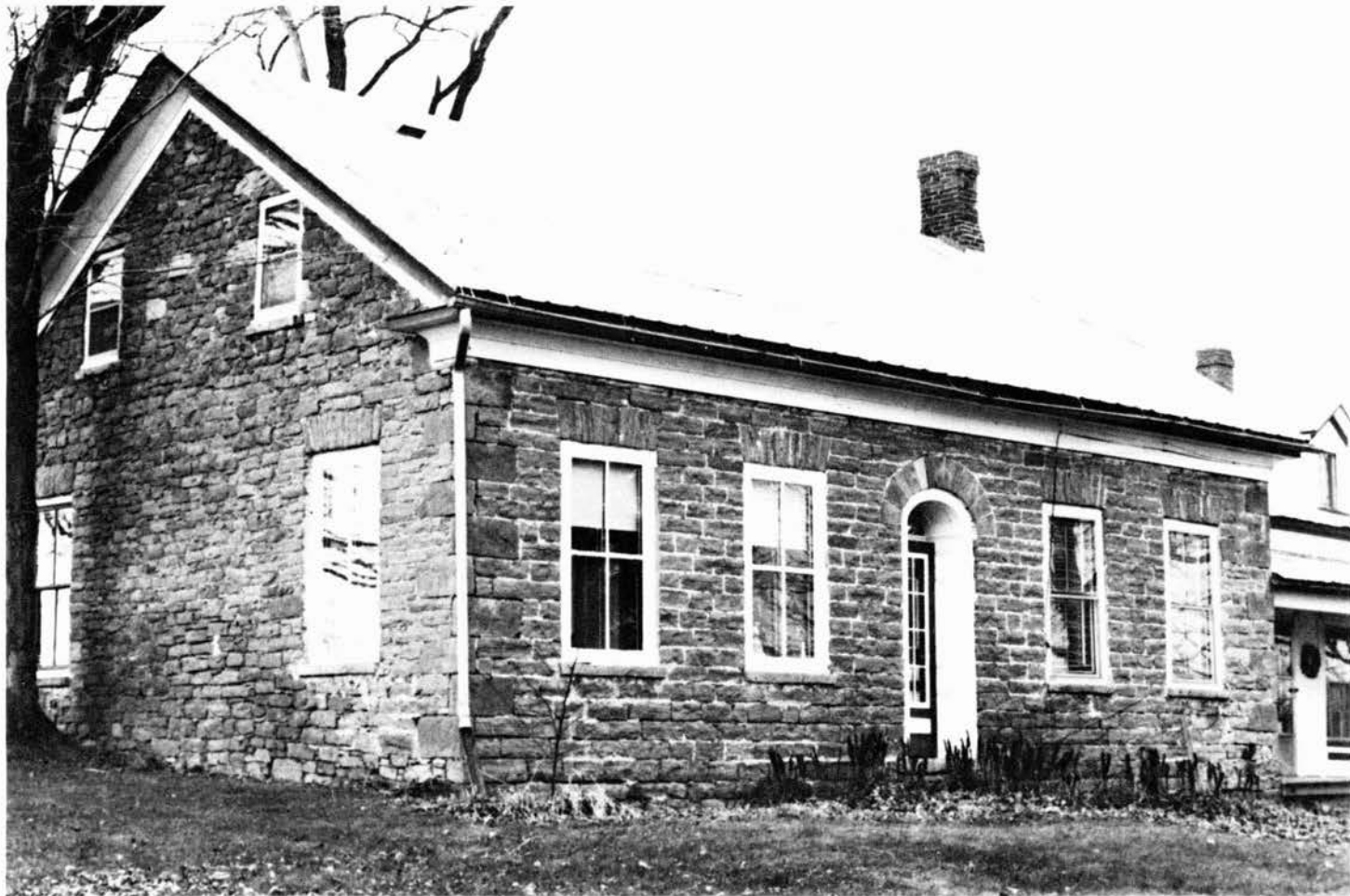
William Day home on Buck Road. Evidence of more sophisticated construction methods and influence of architecture style: semi-circular, fan shaped doorway; smooth, regular courses of stonework on front; and rougher, more random treatment on side. (Photo courtesy of Pauline Tedford)
