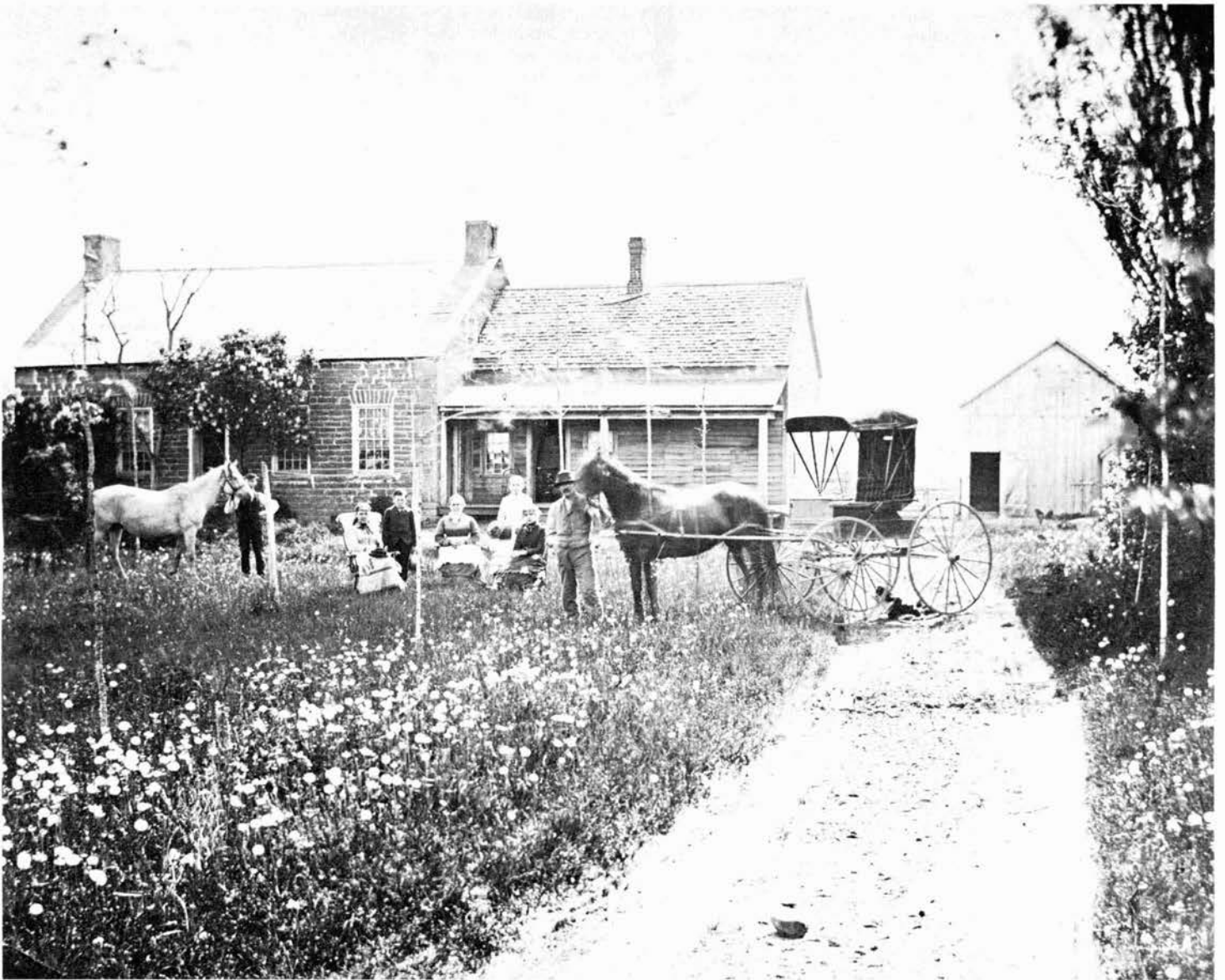
A simple stone cottage in the Chipman area settled by Scot families in the early nineteenth century. This early photograph shows the basic stone structure with a frame construction wing and porch. (Photo courtesy of Pauline Tedford)
