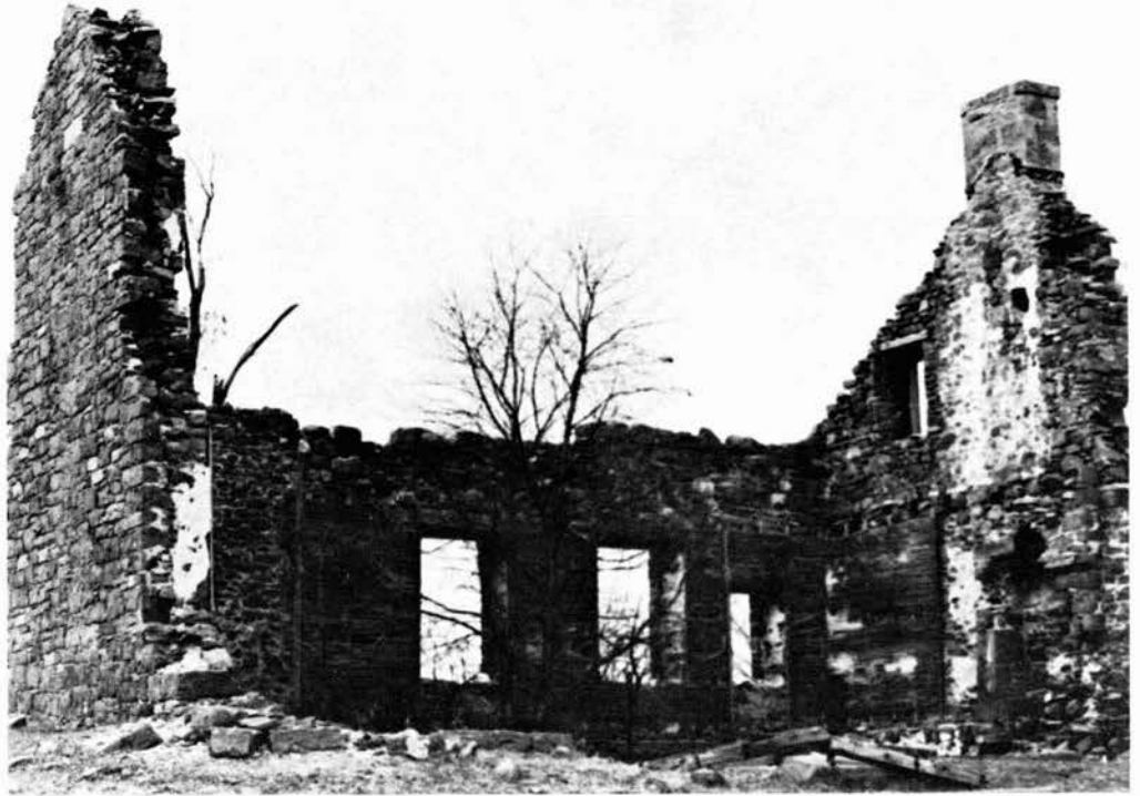
Ruin of a stone cottage on Buck Road, showing the inclusion of the fireplace into the gable end walls and the thick stone walls. (Photo courtesy of Pauline Tedford)
