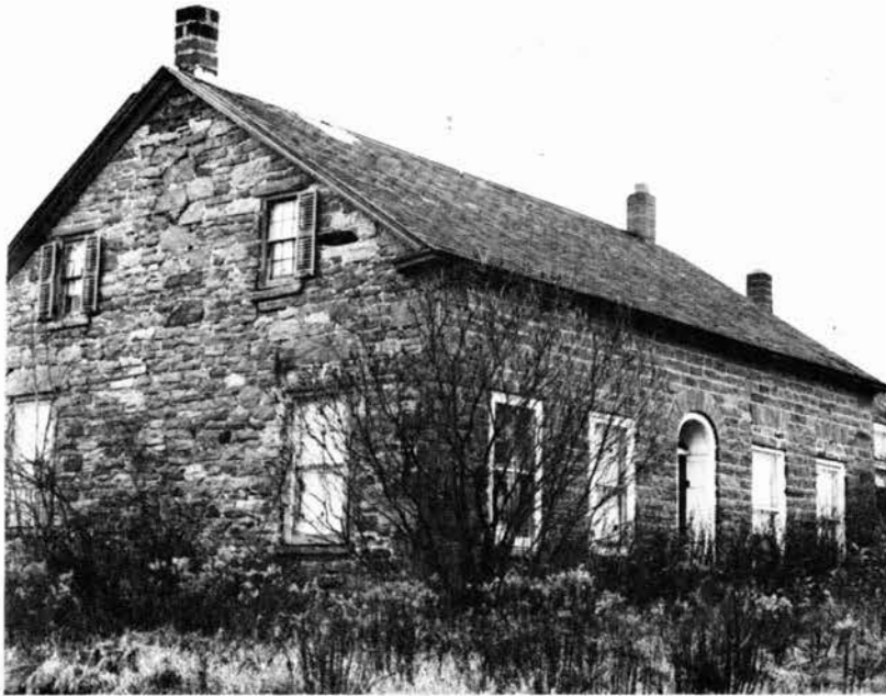
Rookey house at Chipman Corners. Coarse rubble on gable ends, smooth cut on facade, frame construction wing. (Photo courtesy of Pauline Tedford)
