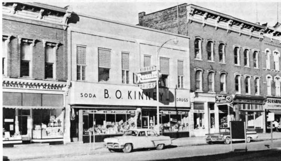
The Kinney Drug Store, with the familiar Rexall sign, as it appeared for thirty years. The 1960 and the 1977 expansions have taken in the two stores in the building to the right. (Photo courtesy of Kinney Drugs).
