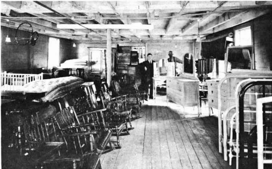
Interior of Mayer Sperling's first store, Riverside Drive, Canton.
