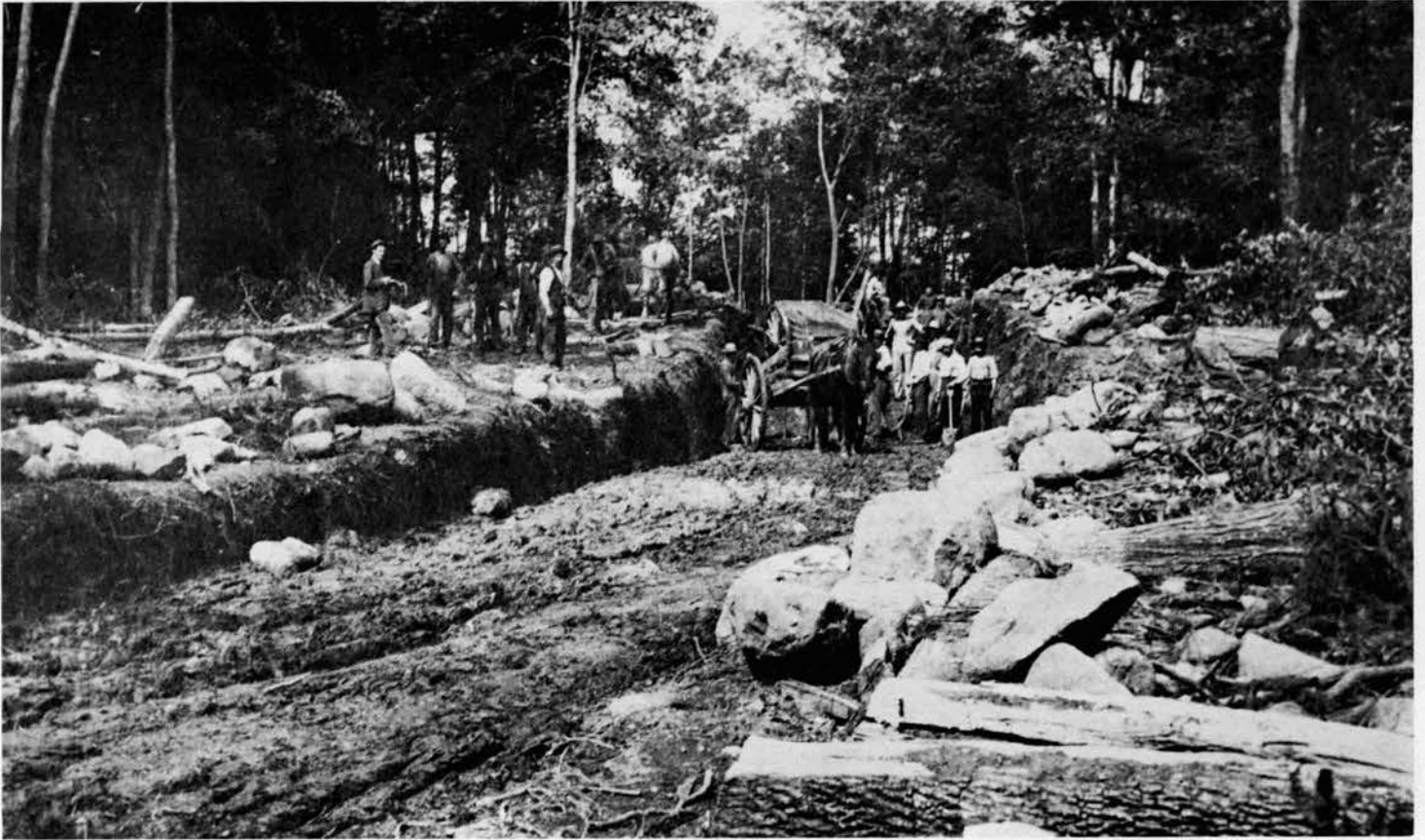
August 14, 1897 — Cutting through ridge in back of canal for the railroad which runs along canal.
