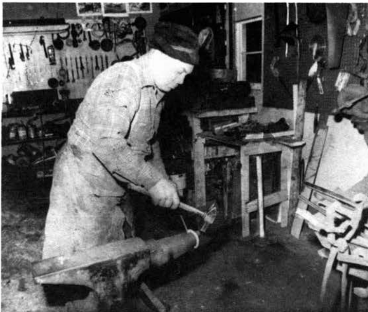
Left: Eli Tracy demonstrates the use of the anvil in making the round handle of a stove poker;
