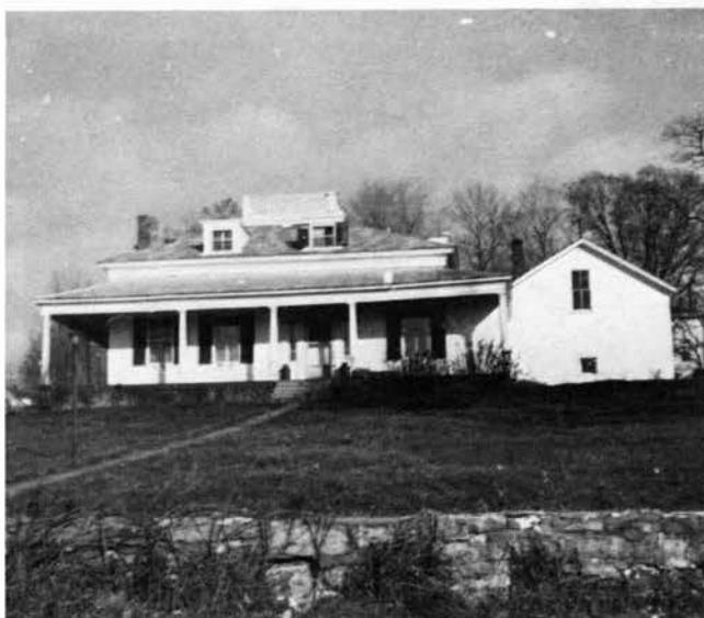
In 1818 Church went to Morristown to survey the area into lots at the request of Col. Nathan Ford. Among the houses believed to have been built by Church is the John Hooker House built for one of Parish's Great Lakes ship captains.
