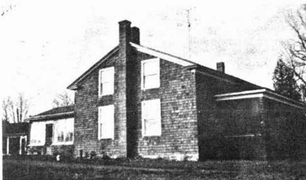
This house, believed to be the oldest still standing in Norfolk village, was built by Phineas Atwater.
