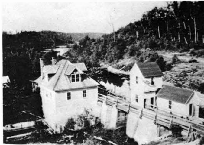
Second dam in the Bog by Low. Power House and tail race visible.
