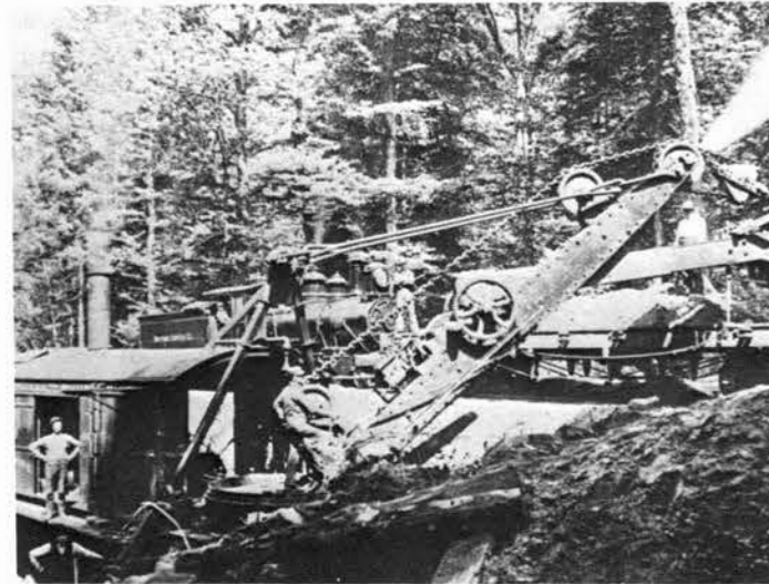
Excavating footings at first dam.
