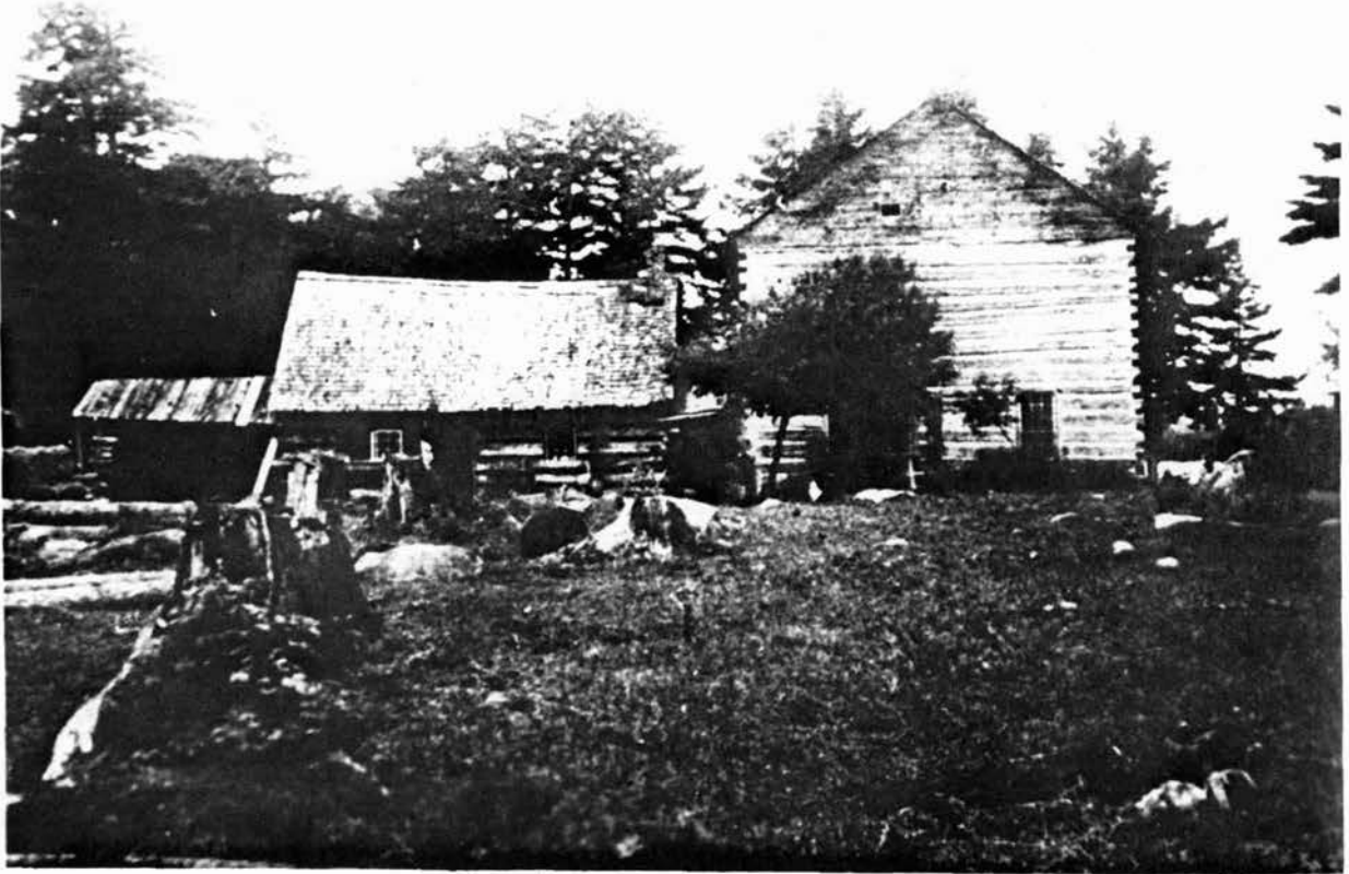
The Old Log Hotel, rear view.
